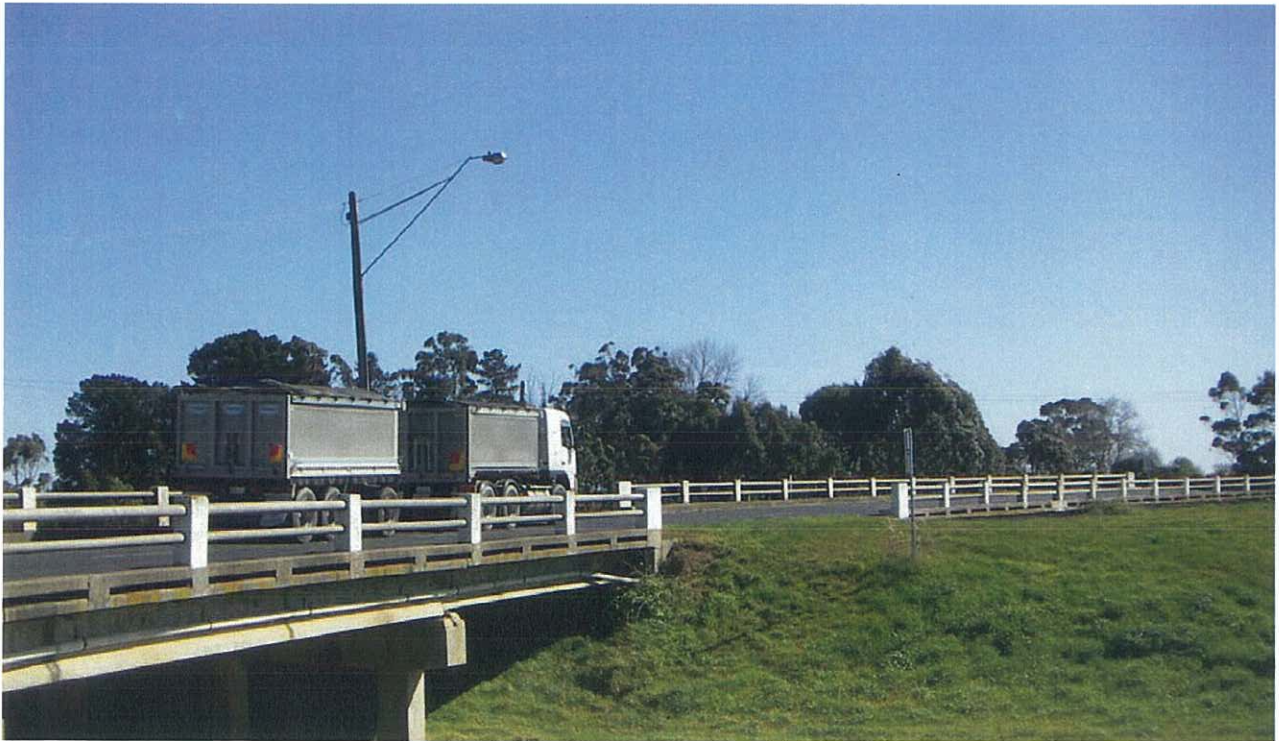
Above: Looking north along Healesville-Koo Wee Rup Road from Bunyip River
