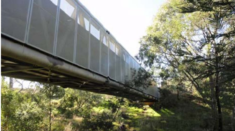
Figure 5 Typical pipe bridge post construction
