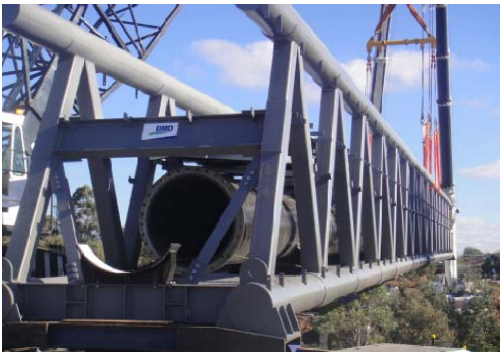
Figure 4 Typical pipe bridge during construction
