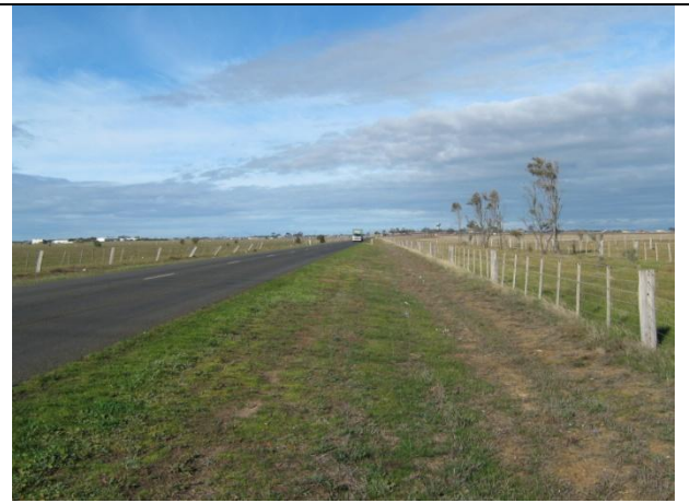
Plate 73: Disturbed alignment along Tarneit Road, facing south.
