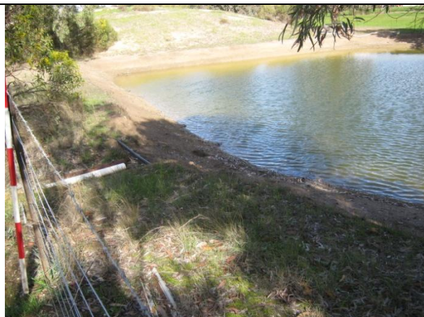
Plate 17: Disturbance due to excavation of a dam along the alignment.
