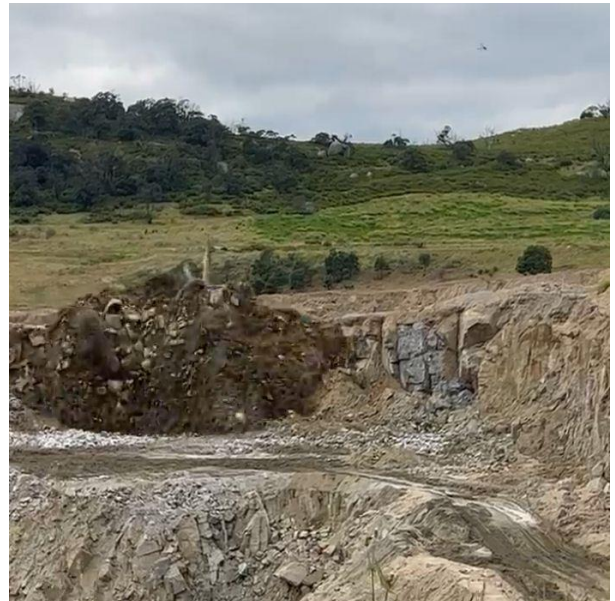
Fig 6b – Blast fired 04/11/2022
