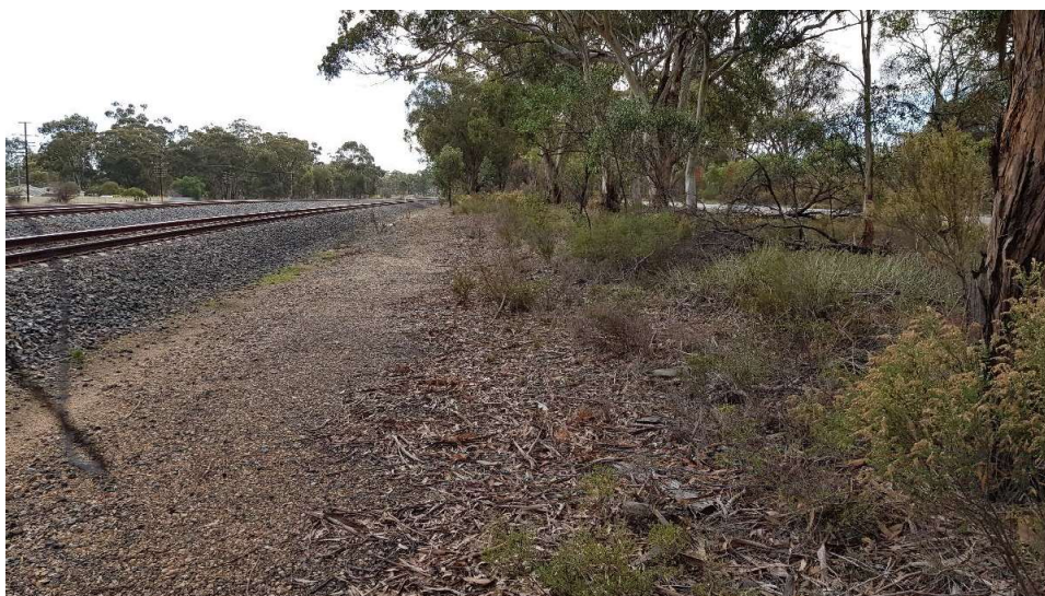
Figure 4 GBGW at Track Slew Investigation Area I between Seymour and Mangalore
