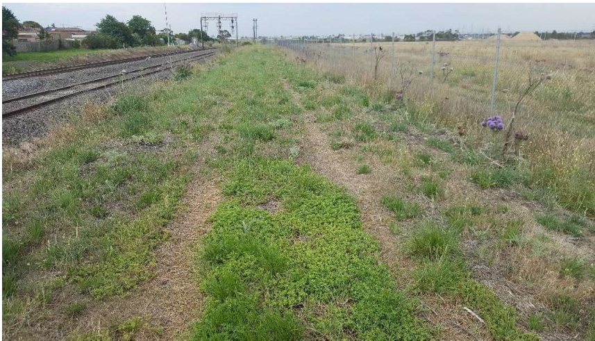
Figure 1 Rail Reserve at Keilor Park Drive Overbridge (Keilor East)
