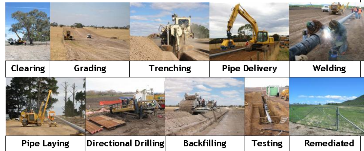
Figure 3 Typical pipeline construction activities
