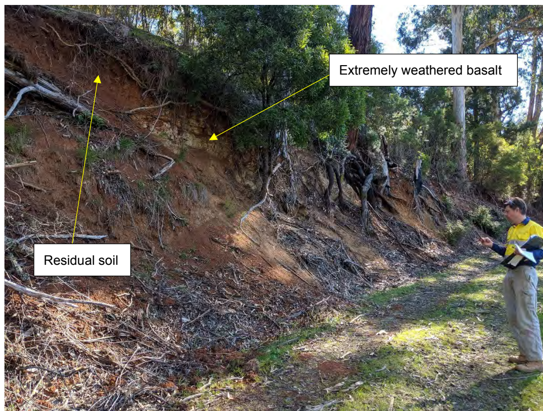
Cutting exposed about 100 m to the north of WTG46
