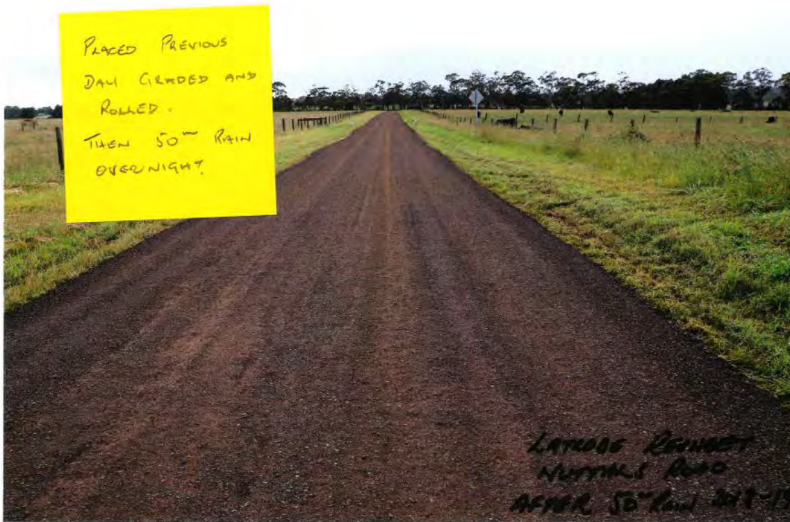
40 mm Non-Descript Crushed Rock resheet. Photo provided by Ross Kennedy
