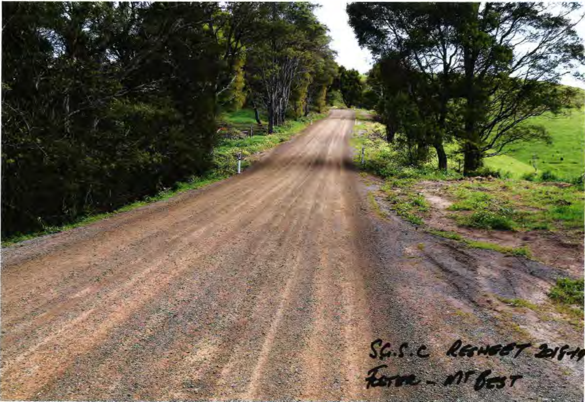
40 mm Non-Descript Crushed Rock 'resheet mix'. Photo provided by Ross Kennedy
