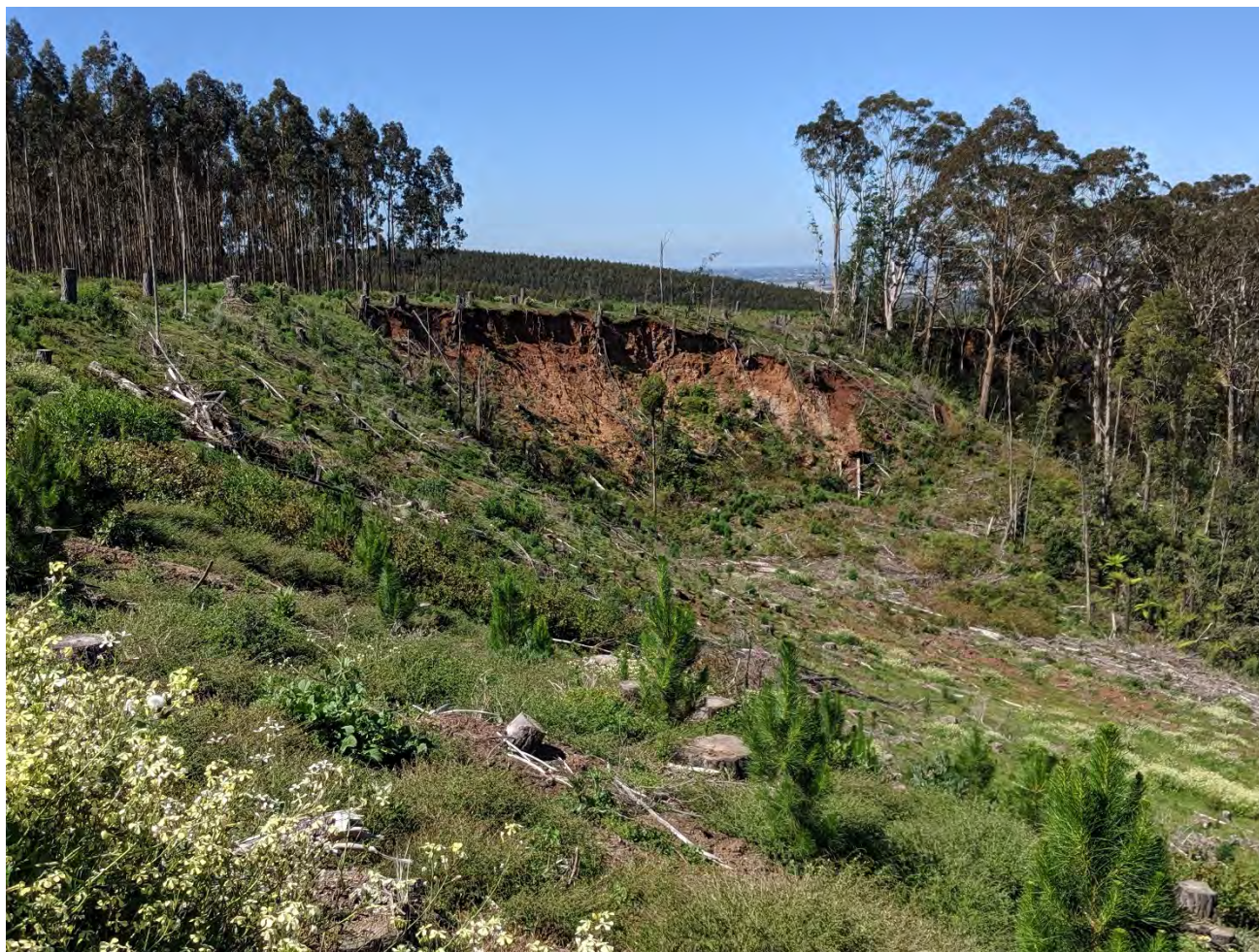
Plate 5: Example of recent landslide, traverse between WTG 8 and WTG 9
