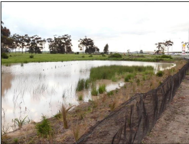
Plate 3. An example of fencing designed to prevent frog passage beyond the wetland/waterway
