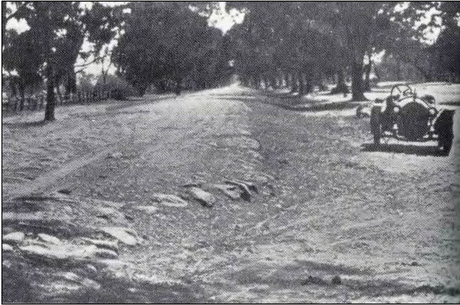
Figure 2-4: The Hume Highway in the days when it was known as Sydney Road. The road's poor condition is evident by the exposed foundation stones, 1914 (Anderson 1994).
