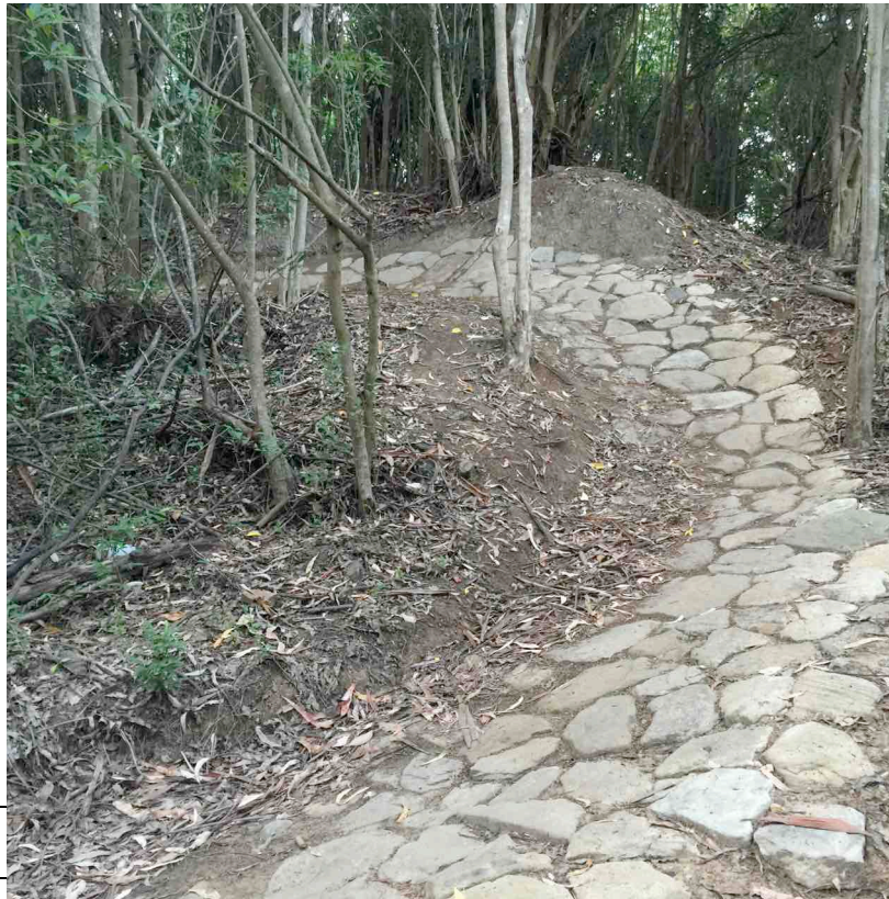
Rock armouring example image- Hornsby, NSW
