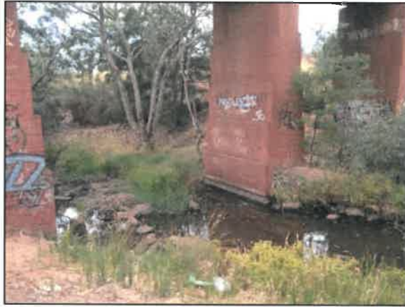
Plate 15 Bridge crossing at Toolern Creek
