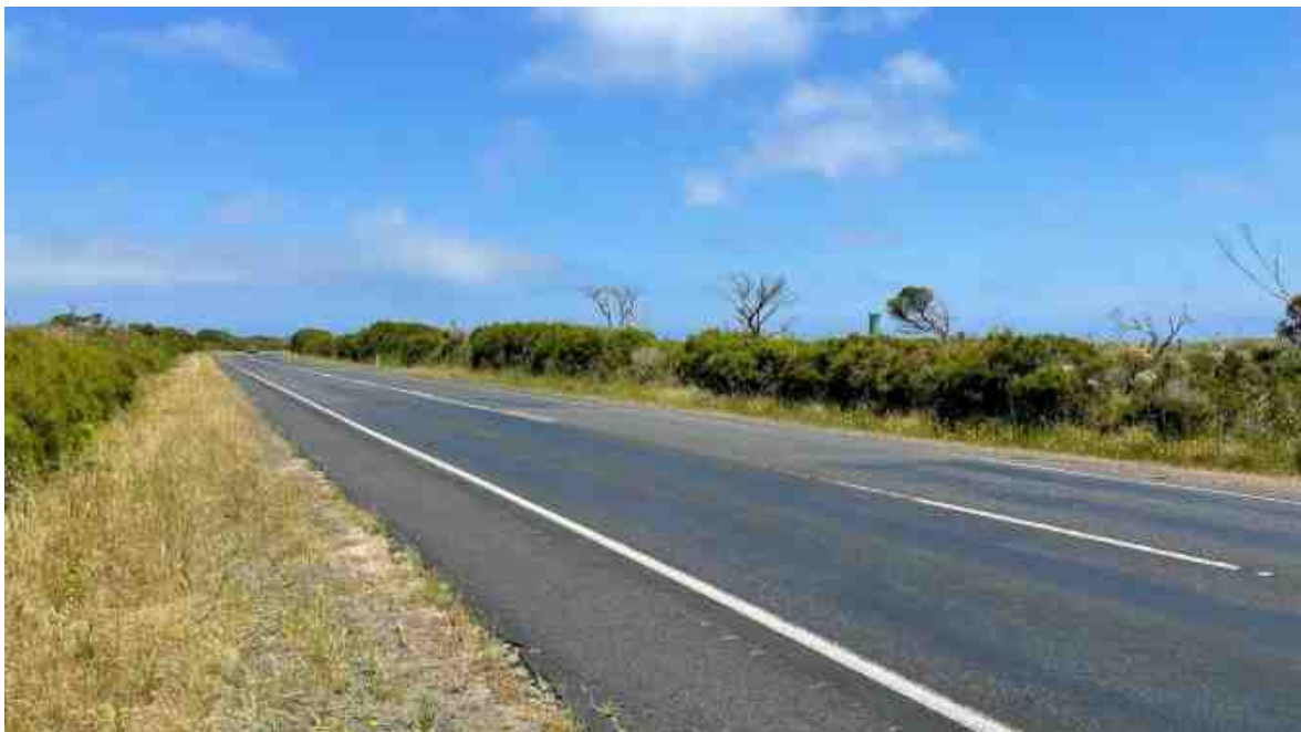
Figure 10: Cape Paterson Road on approach to Cape Paterson settlement, with remnant roadside vegetation.
