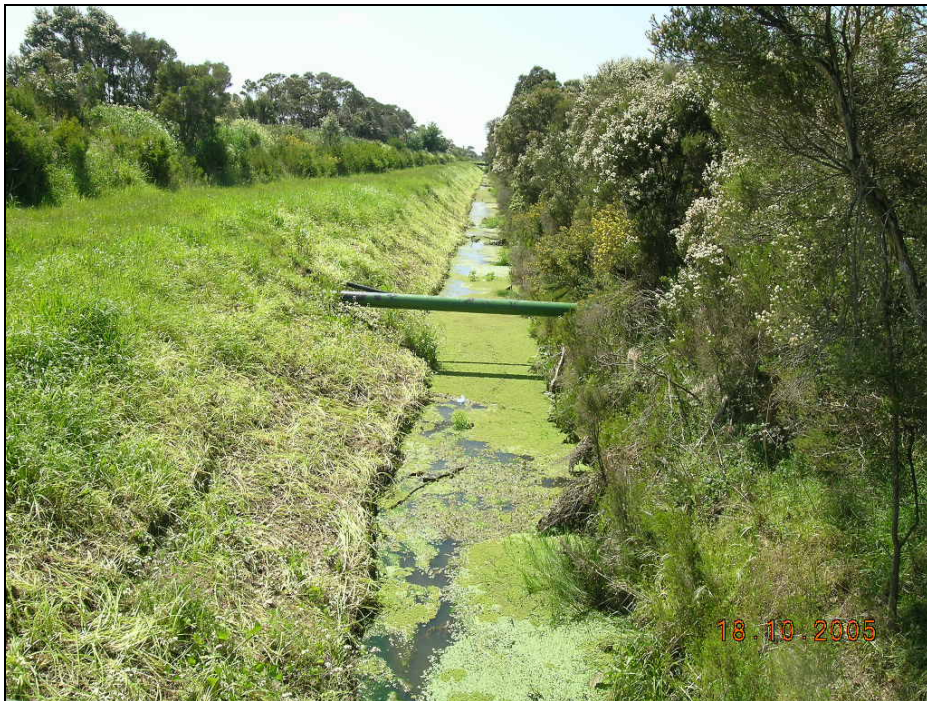
Photograph 6. Town Drain (Site 15).
