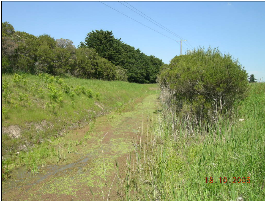
Photograph 3. Healesville Koo Wee Rup Road Drain (Site 5).
