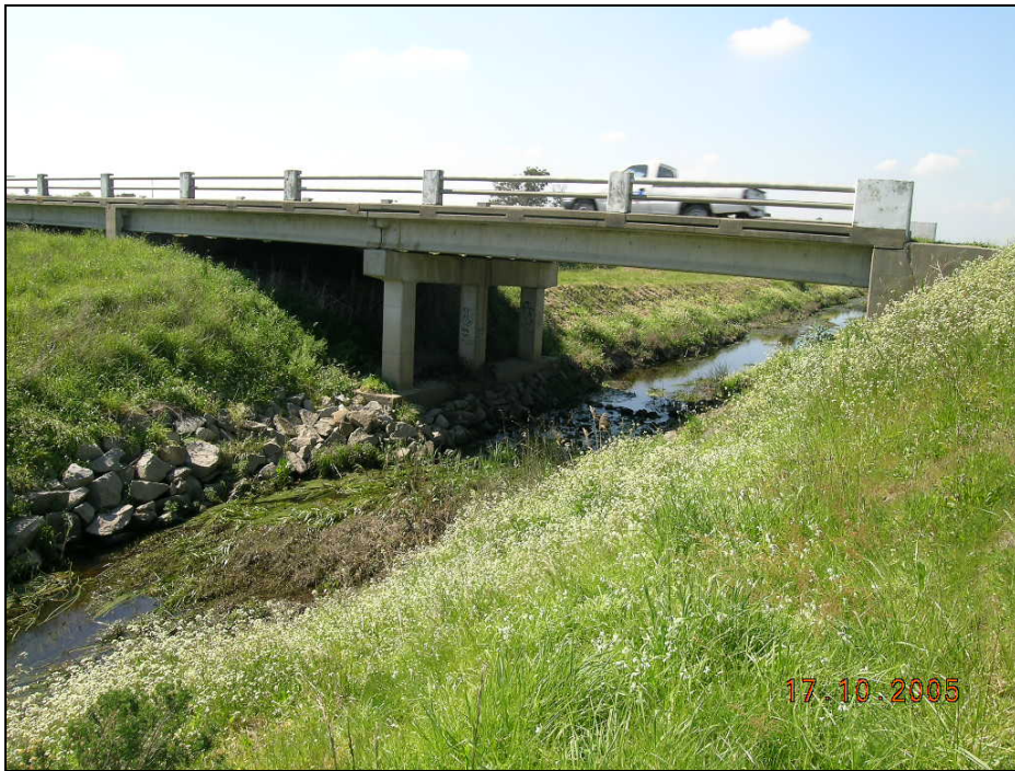
Photograph 5. Nine Mile Road Drain (Site 13).
