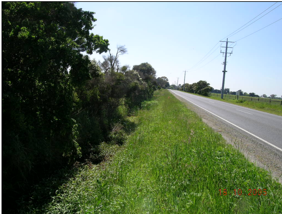
Photograph 8. Rossiter Road Drain (Site 19).
