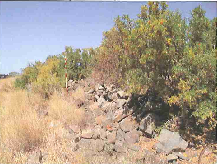
9. Drystone wall, looking west
