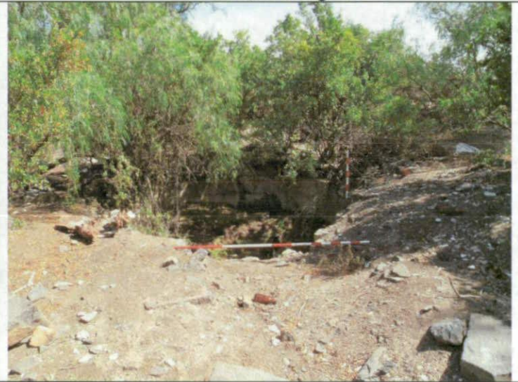
3. Blue stone lined cistern, looking west
