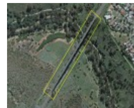
Albion Viaduct Extent Aerial June 2021
