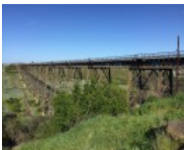
RAIL BRIDGE (ALBION VIADUCT) September 2016
