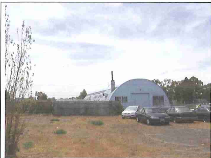
1. Nissen type building to the north of the site, looking north
