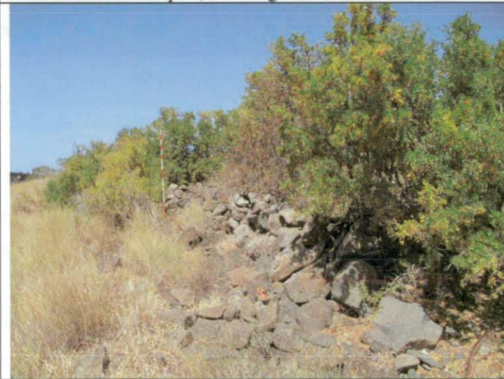
9. Drystone wall, looking west
