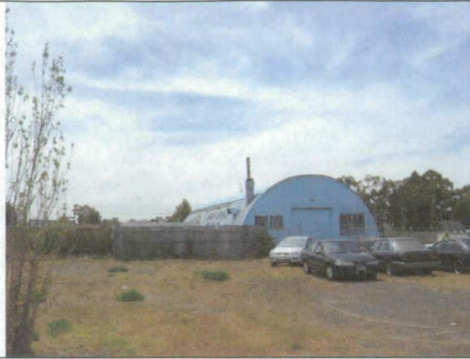
1. Nissen type building to the north of the site, looking north
