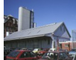
john darling & son flour mill albion delivery building
