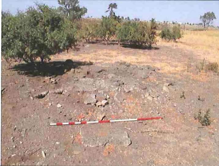
6. Concrete foundation, looking south west
