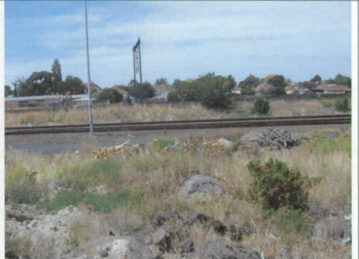
3. Piled material at the south eastern end of the site, looking east
