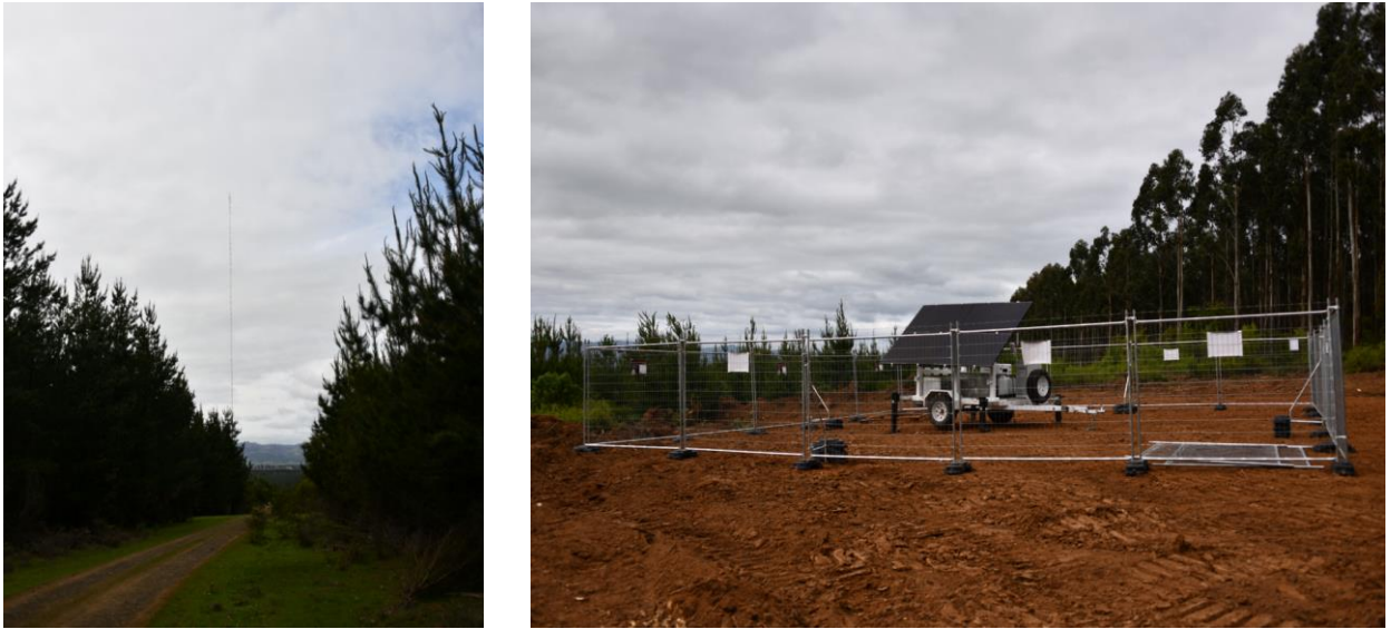
Figure 3-7 Existing meteorological mast and LIDAR units
