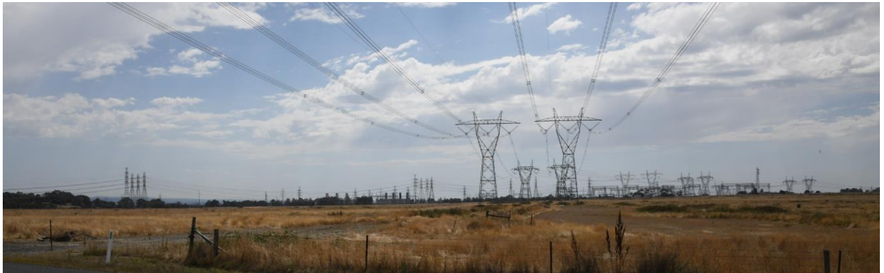
Figure 6-9: Landscape Unit 3 – Industrial/Mining example (Transmission Line)
