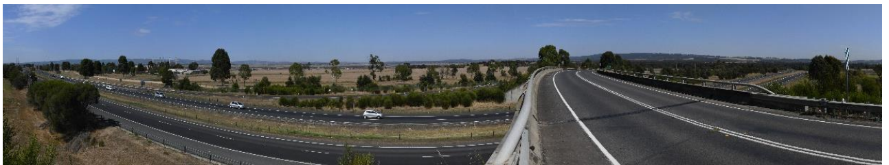
Figure 8-7: Viewpoint M2 – Existing view looking south west
