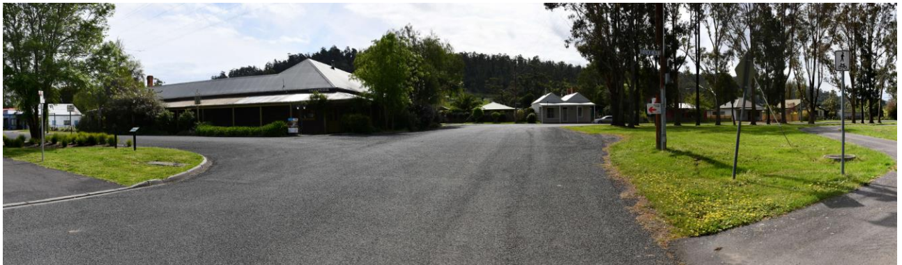
Figure 8-77 View looking southwest to northwest
