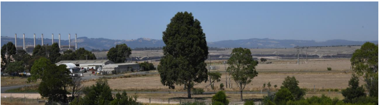
Figure 6-7: Landscape Unit 3 – Industrial/Mining example (Yallourn Power Station)
