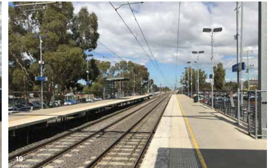
19 Keilor Plains Station platforms
