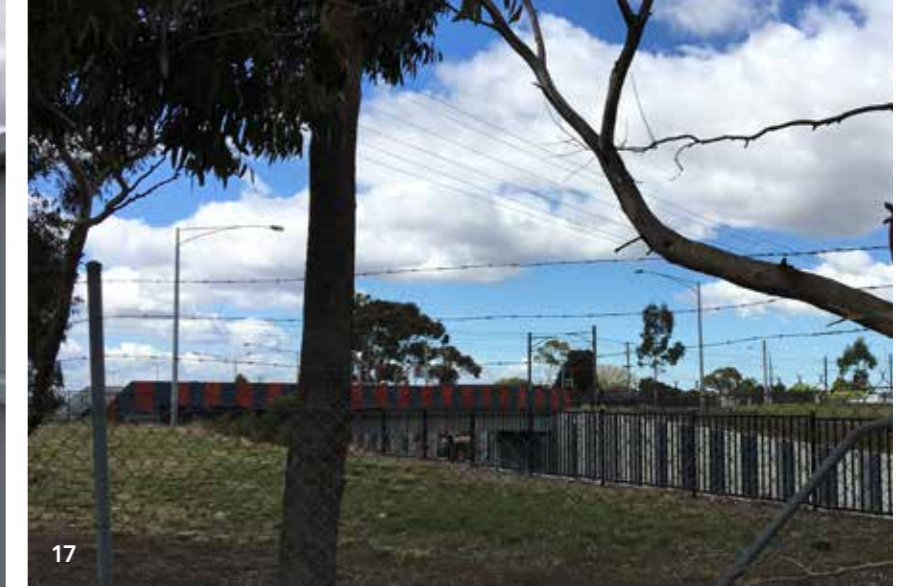
17 Looking south at below grade section of Taylors Road Keilor Plains Station
