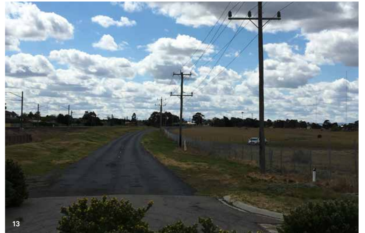
13 Looking north from the end of the discontinued Sydenham Road
