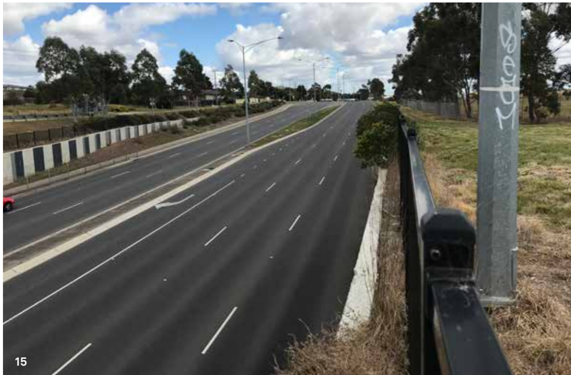
15 Large grade separation/barrier at Taylors Road at south eastern corner of site
