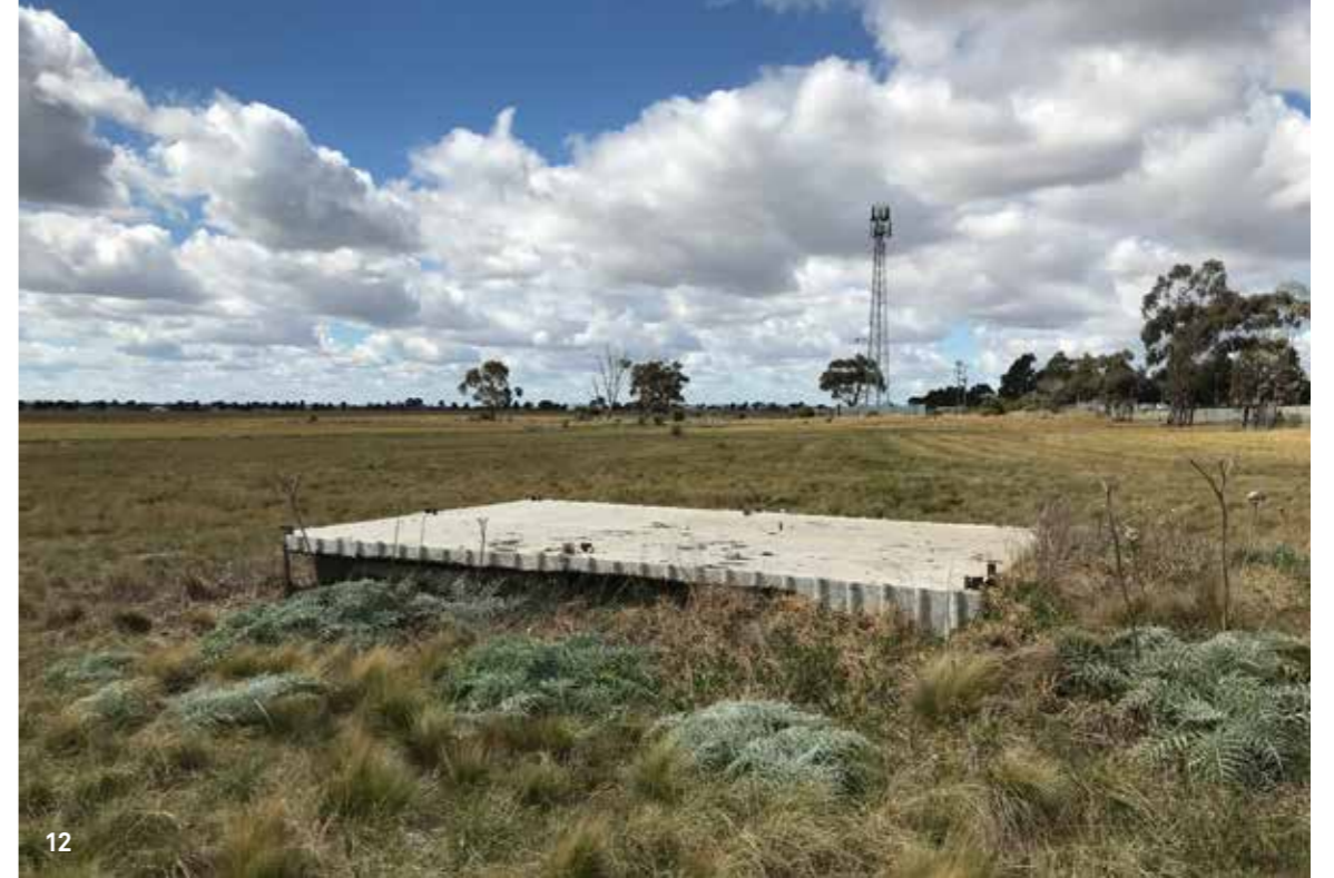
12 Existing concrete base
