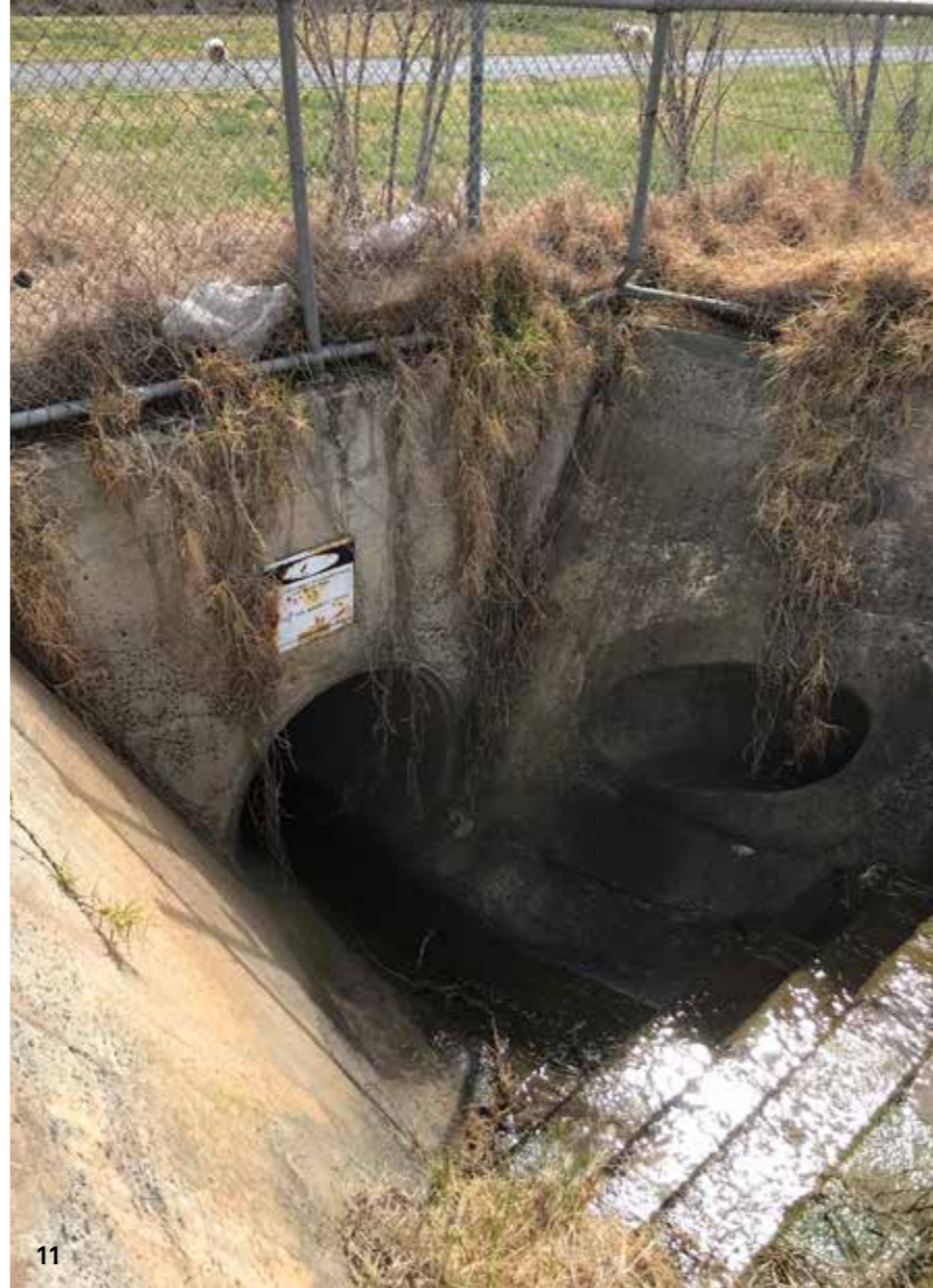
11 Existing underground culvert pipe
