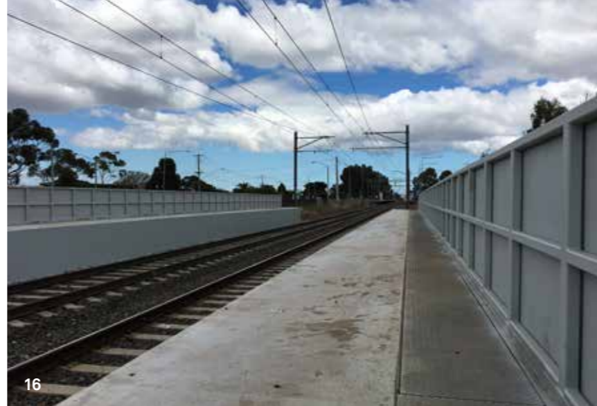
16 Footbridge overpass (no public access) across Taylor Road at south eastern corner of site
