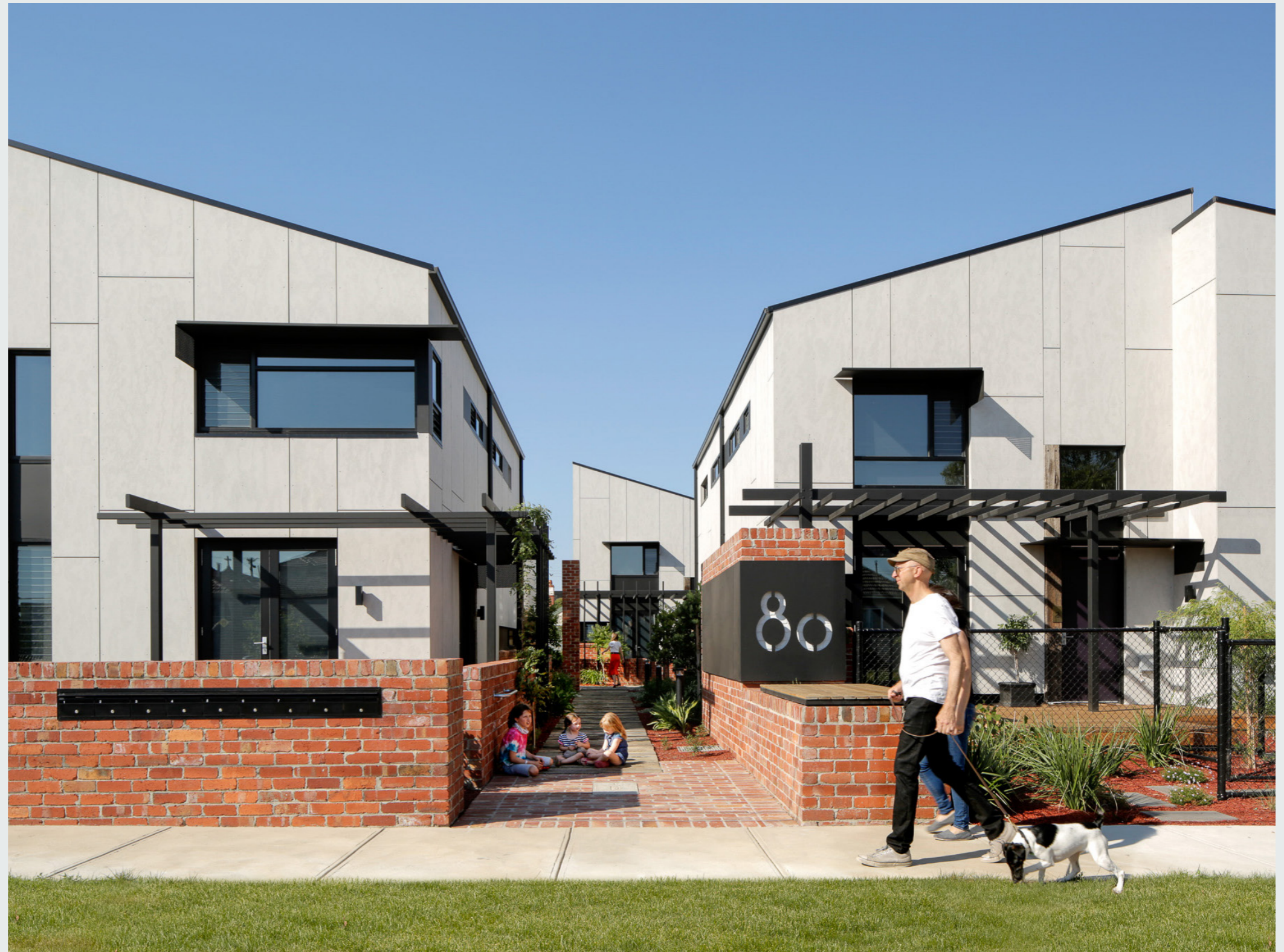
▲ 1.01 Clyde Street Mews, Thornbury VIC - Six Degrees Architects
