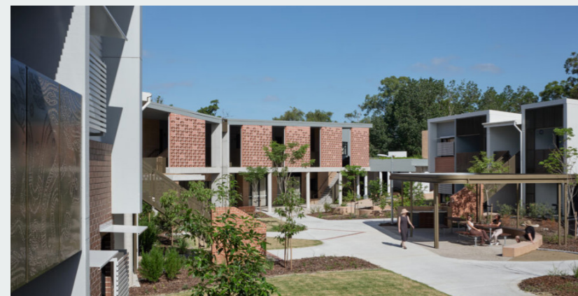
Addressing and enhancing local identity can generate lasting social value. The Mari-Mari-Ba housing development, built on a site with rich cultural and community history, offers support services and communal spaces for residents and visitors. First Nations voices were integrated and culturally appropriate designs achieved. A community hub at the front of the site includes support services, amenities and utility spaces, while the more private and culturally sensitive spaces are located deeper within the site.
