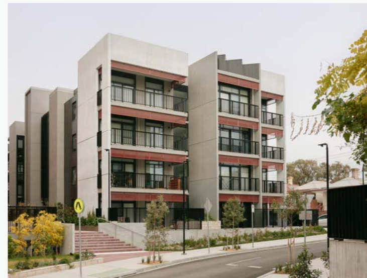
▲ 7.04 Victoria St, Flemington VIC - Architect: Six Degrees Architects, Project Owner: Homes Victoria
