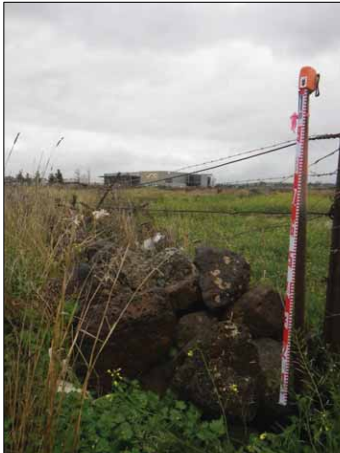
Figure 3-7: Facing south. Image showing the Dry Stone Walls that form part of the newly located dry stone wall Dry Stone Wall 9 (west of Robinsons Road).
