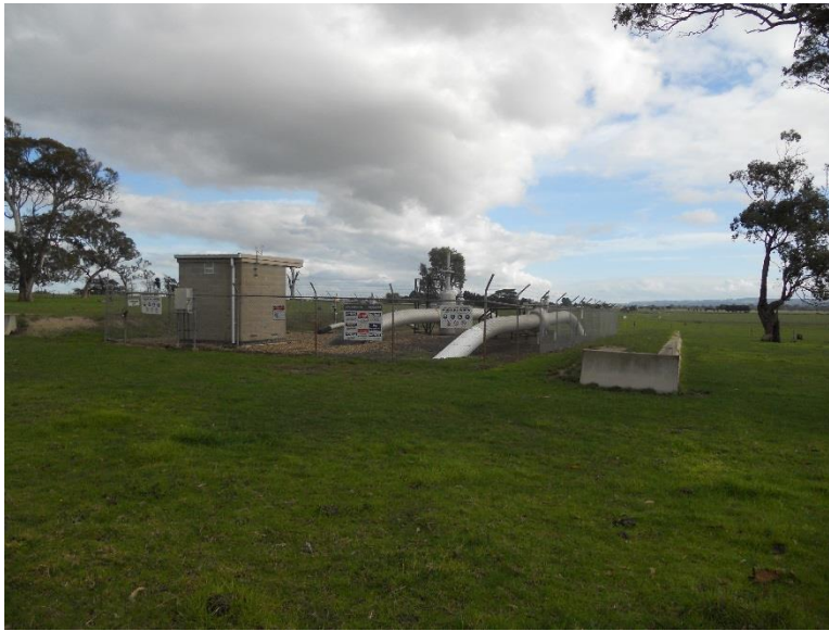
Photo 1 – Existing pipeline valve site
