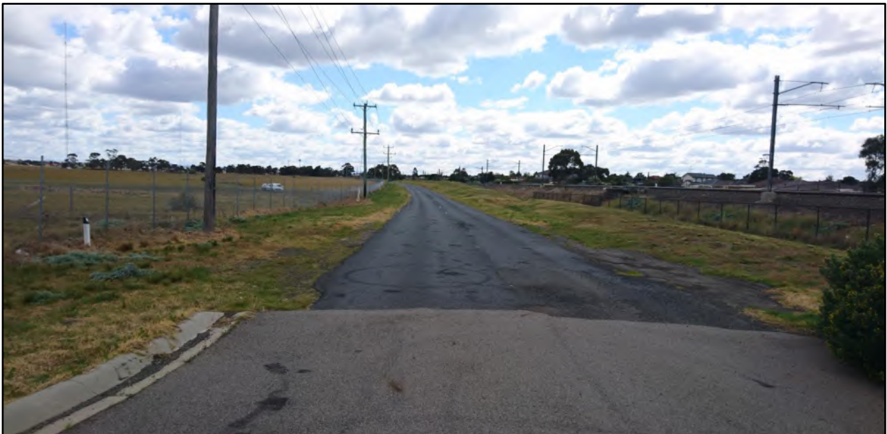
Figure 7 Sydenham Road, looking north from its termination adjacent Taylors Road
