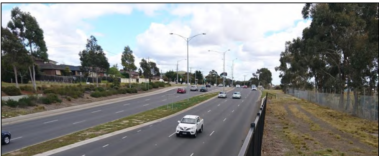
Figure 5 Taylors Road, looking west from the railway line overpass
