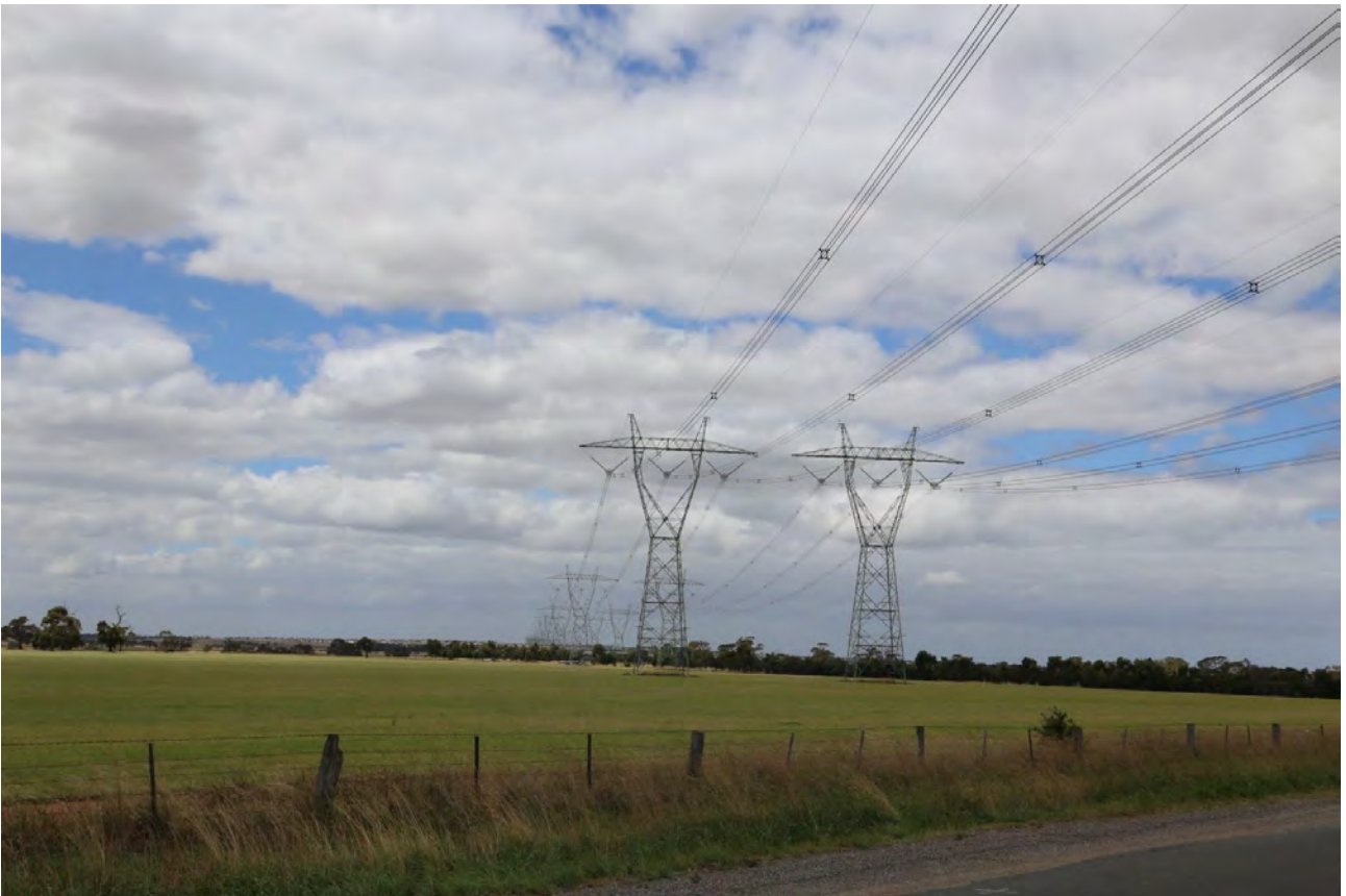
Figure 5 – HV powerlines bisect the Project from southwest to northeast.
