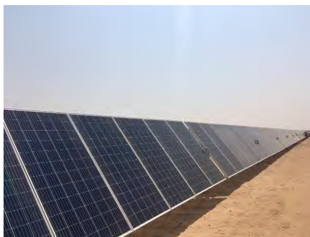
Mounted single-axis bifacial tilting panels.
