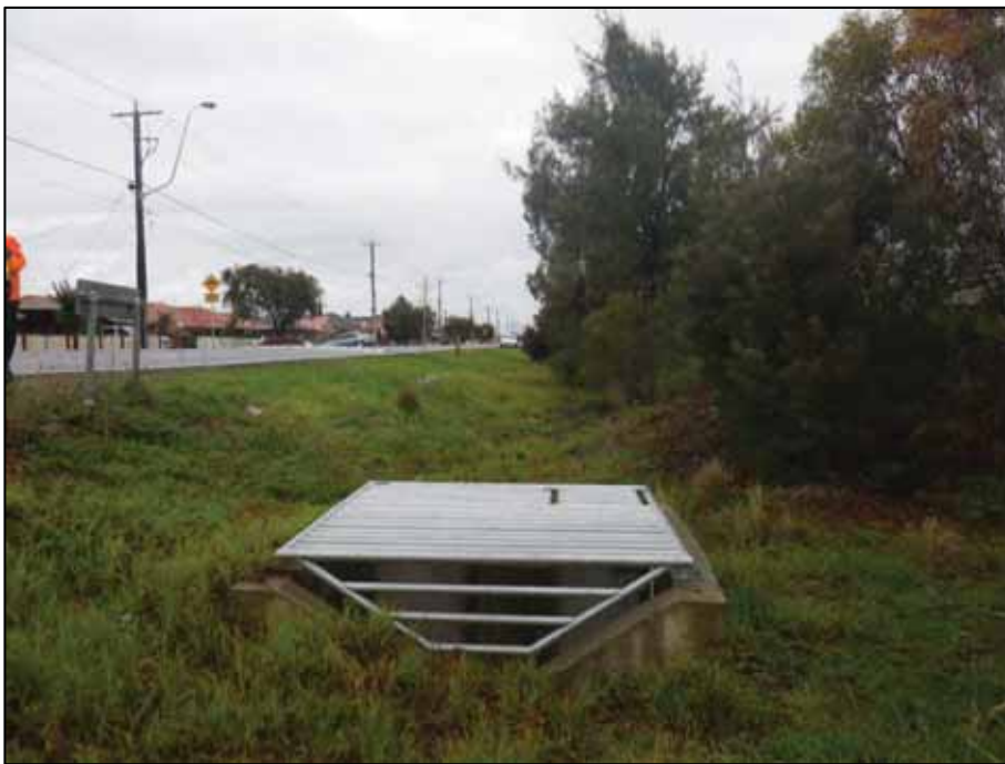
Figure 5-6: Formal swale and drainage within the road verge of Robynsons Road.
