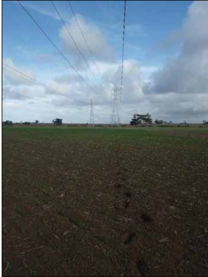
Figure 5-10: View across the activity area where good to excellent ground surface visibility was encountered due to ploughing.
