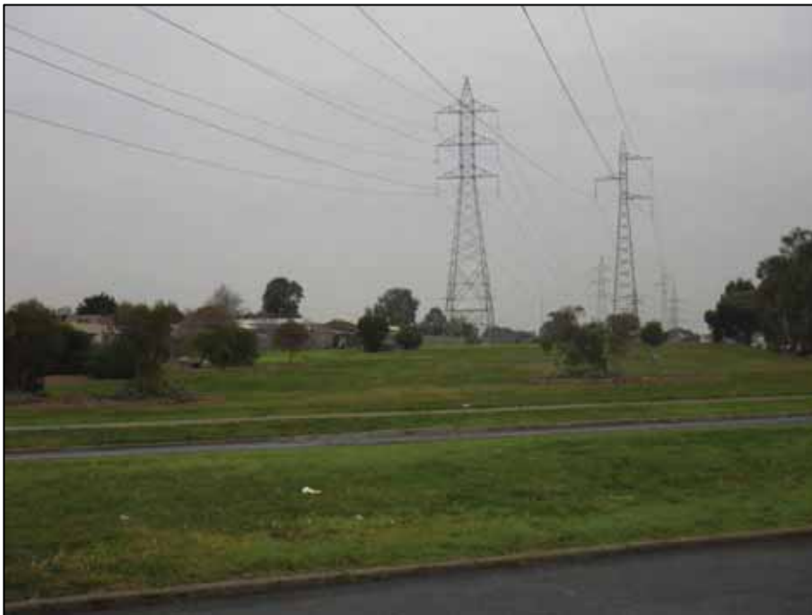
Figure 5-1: General conditions within the powerline easement. View from Neale Road facing north. Residential subdivision is located to the left. A large shopping centre is located to the right.
