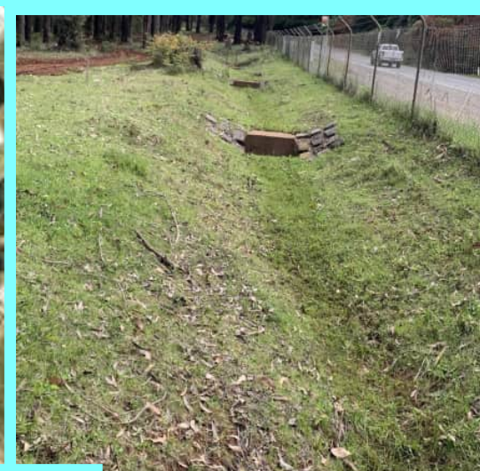
GATE 05 - 06 SWALE DRAIN ADJ FENCE & DRAINAGE CROSSING
