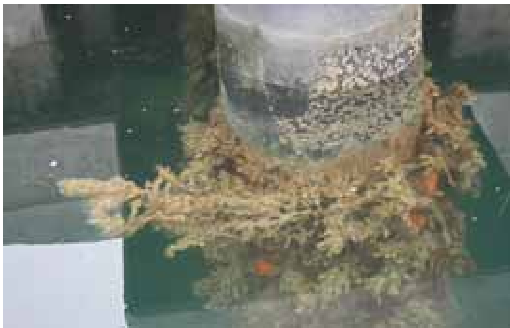
Figure 12: Marine growth evident on the Blairgowrie Marina wavescreeen
