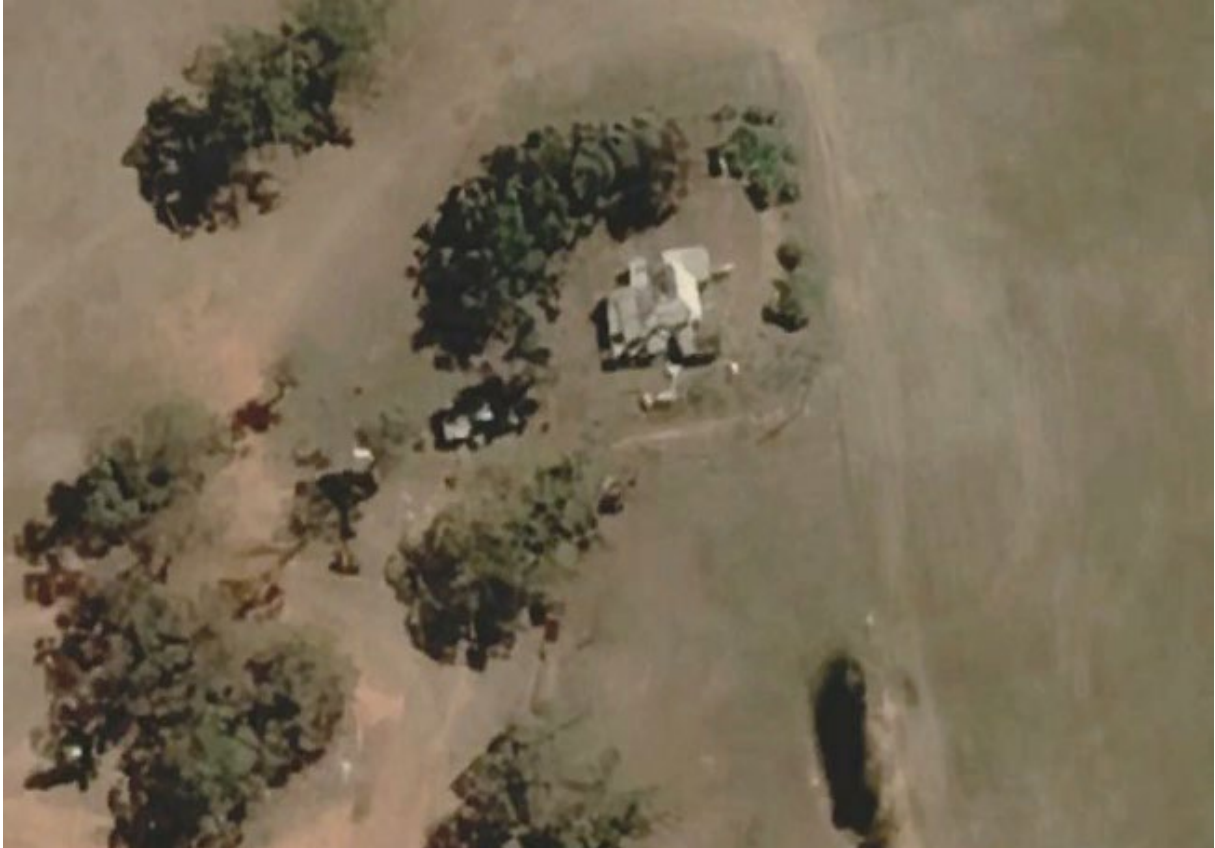
Figure 78 664 North Woodland Road aerial image (sources: Google Earth, March 2021)
