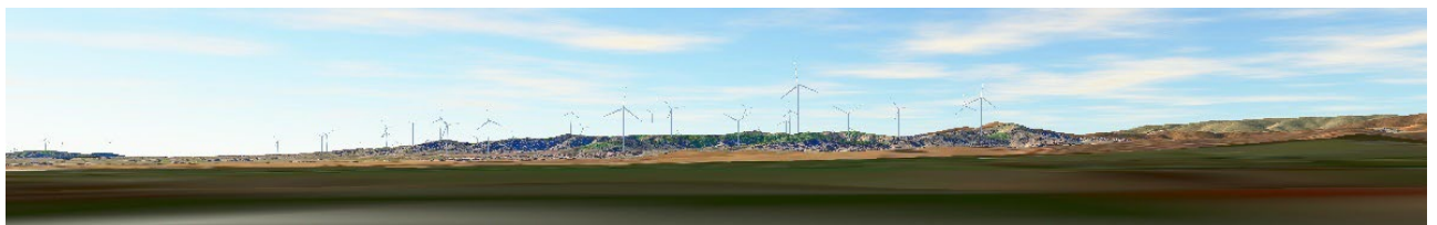
Figure 61 Preliminary render indicative of Project looking north 0 degrees from VP12 (render: Aurecon)
