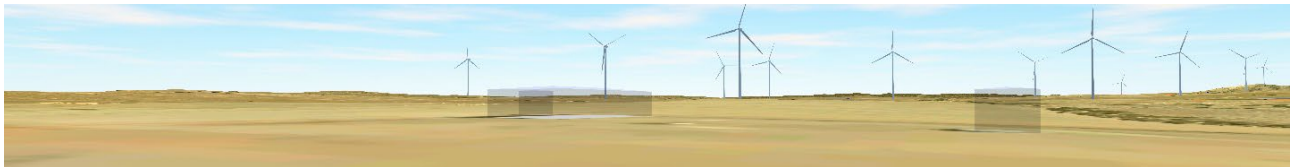
Figure 32 Preliminary render indicative of Project looking northwest 325 degrees from VP2 (render: Aurecon)
