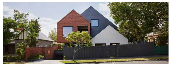
Image credits: Future Homes Program, Department of Transport and Planning, Austin Maynard, Lucent, photographed by Tess Kelly
