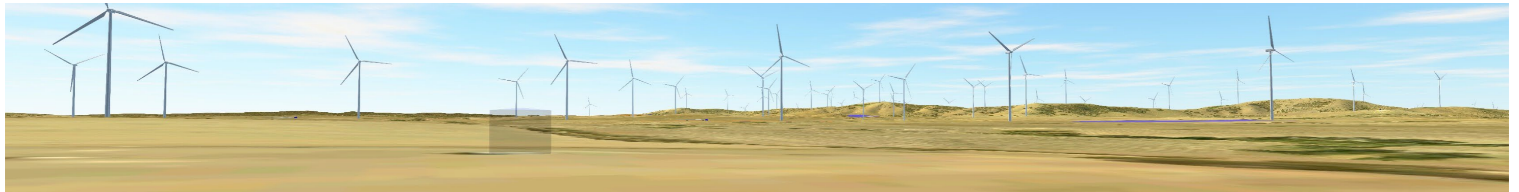
Preliminary render indicative of Project looking north 22 degrees from VP2 (render: Aurecon)
