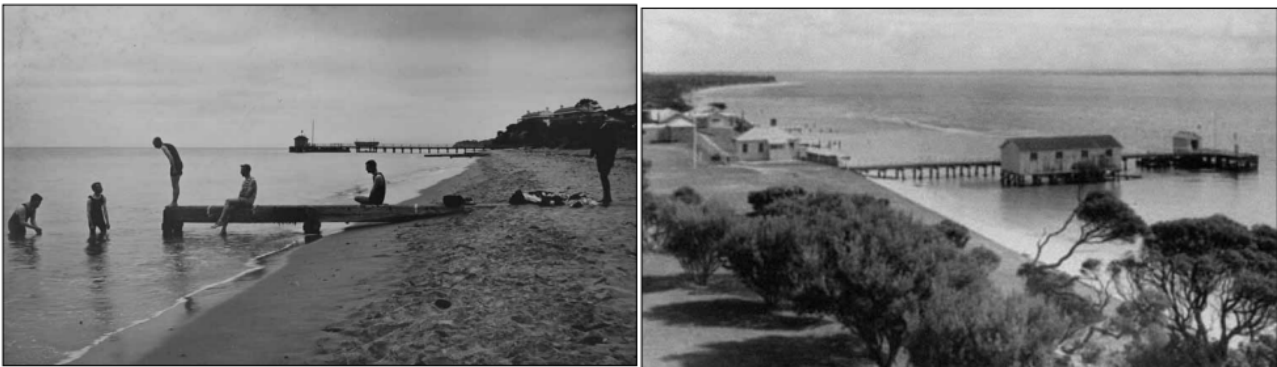
Figure 4.9 Panel A: Wide beach at old storm water outlet pipe 1973. Panel B: No high-tide beach shoreward of seawall 1957. Images: (Bird, 2011)
