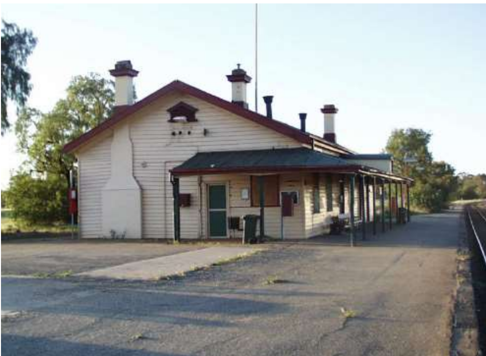
Plate 22 Murchison East Railway Station (Allom Lovell & Associates, 2004)
