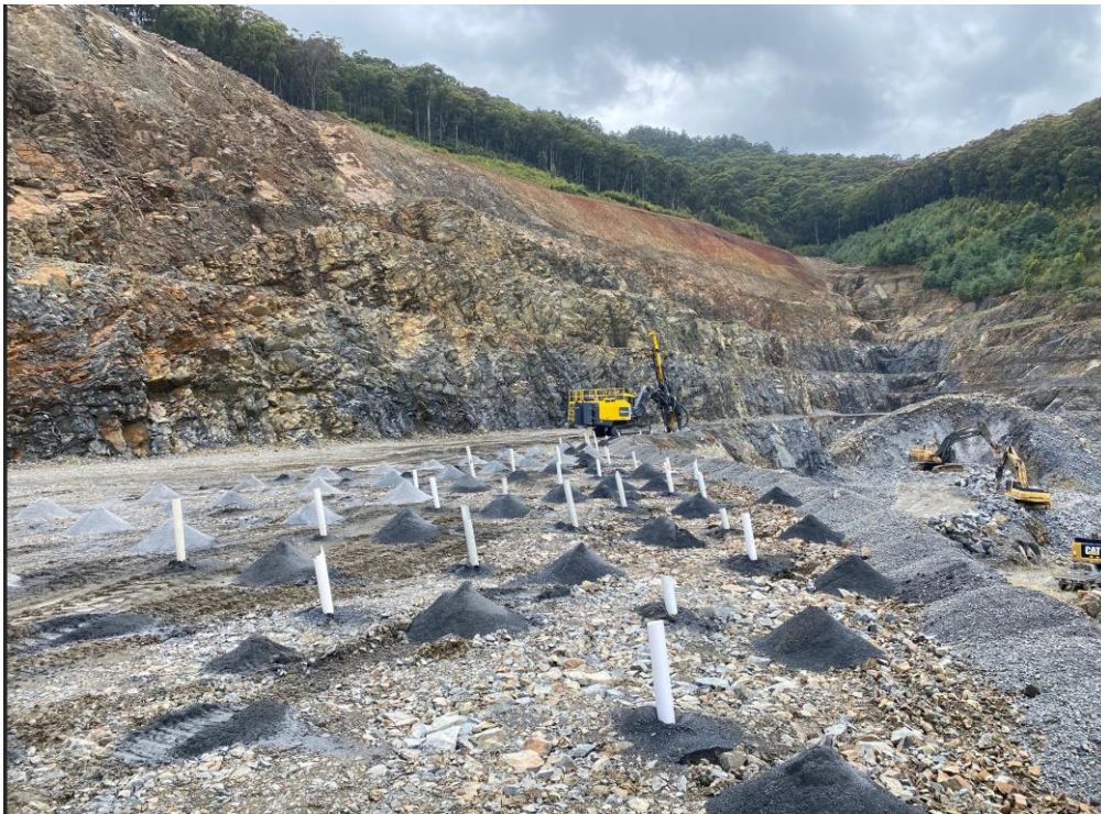
PLATE 8.1 WA375 Blasting Drillhole Layout (courtesy DPQ, 2023)
