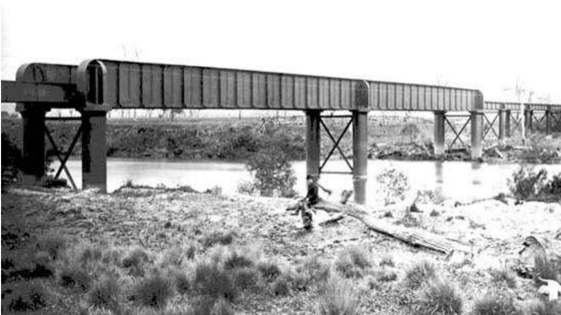
Plate 8 Goulburn River bridge (Public Record Office Victoria)
