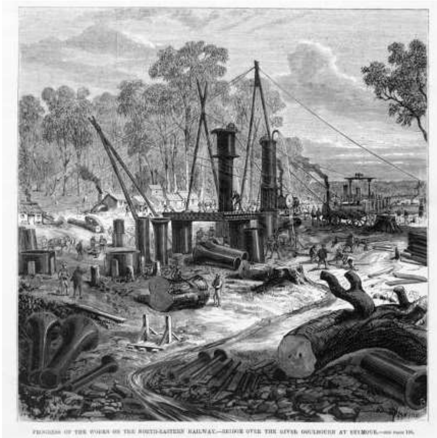
Plate 4 Progress of works on the north-eastern railway bridge over the River Goulburn at Seymour. (Calvert, 1871)
