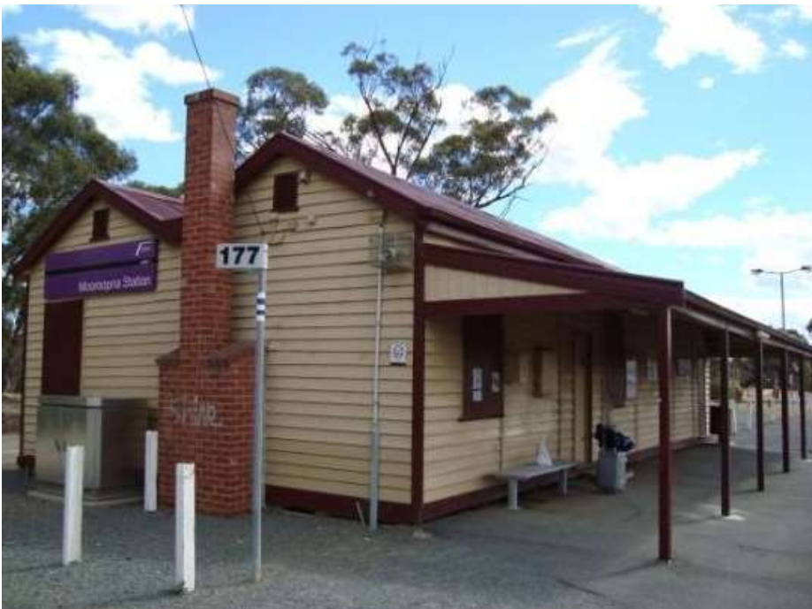
Plate 20 Mooroopna Railway Station, prior to the 2018 fire (Department of Transport, 2018)
