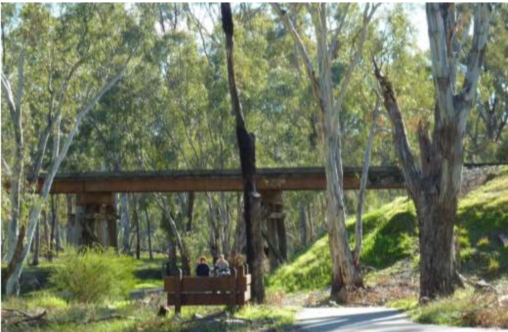
Plate 17 Broken River Railway Bridge (CycleLifeHQ, 2019)
