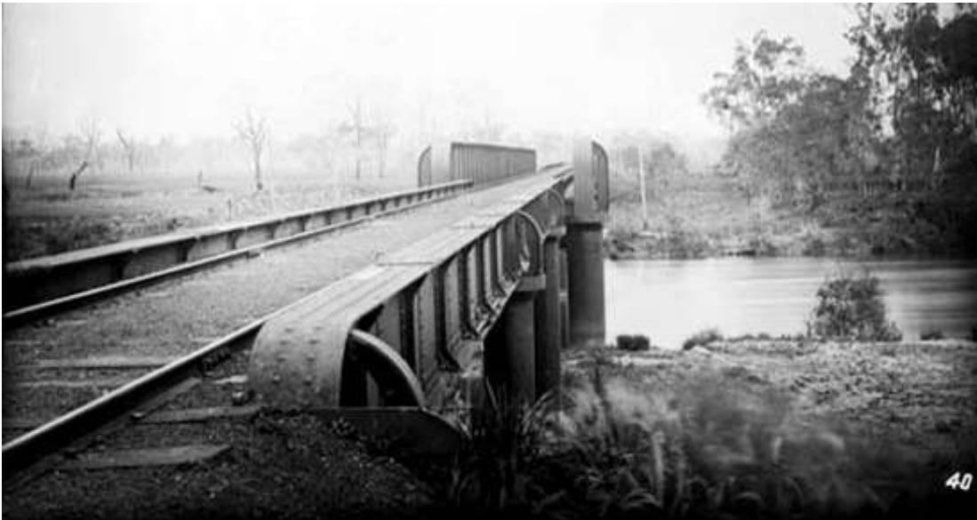
Plate 7 Goulburn River bridge (Public Record Office Victoria)
