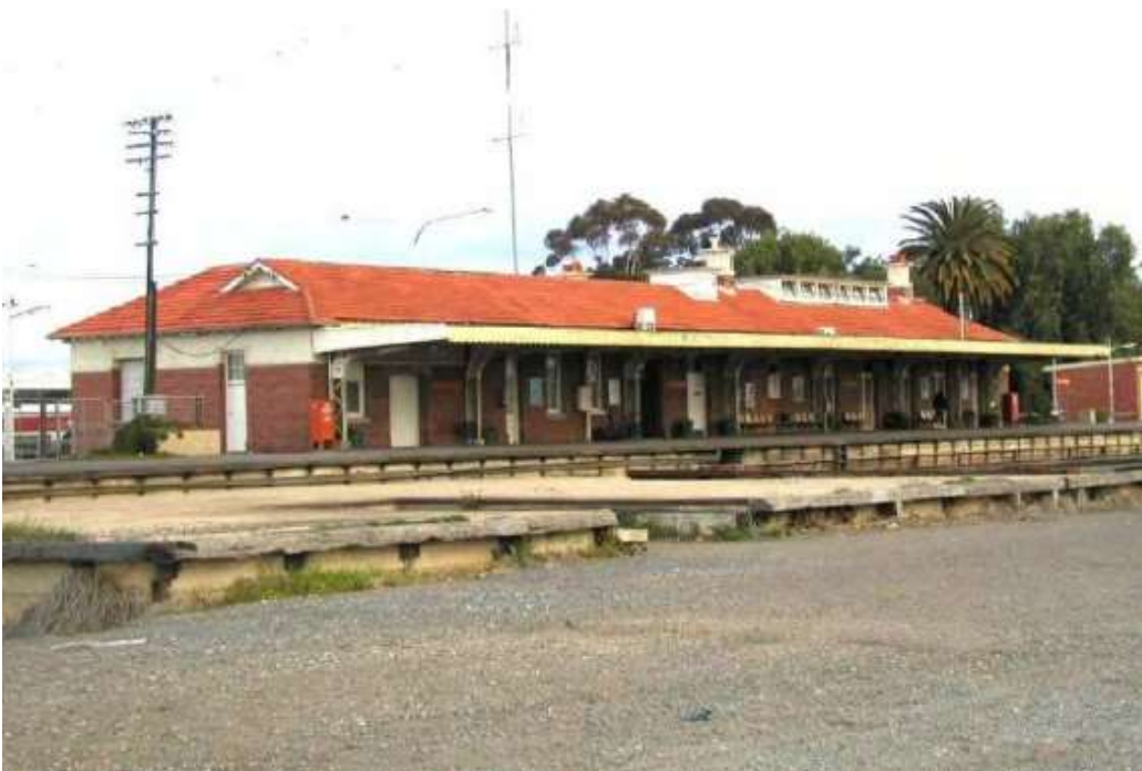
Plate 15 Shepparton Railway Station (Allom Lovell & Associates, 2004)
