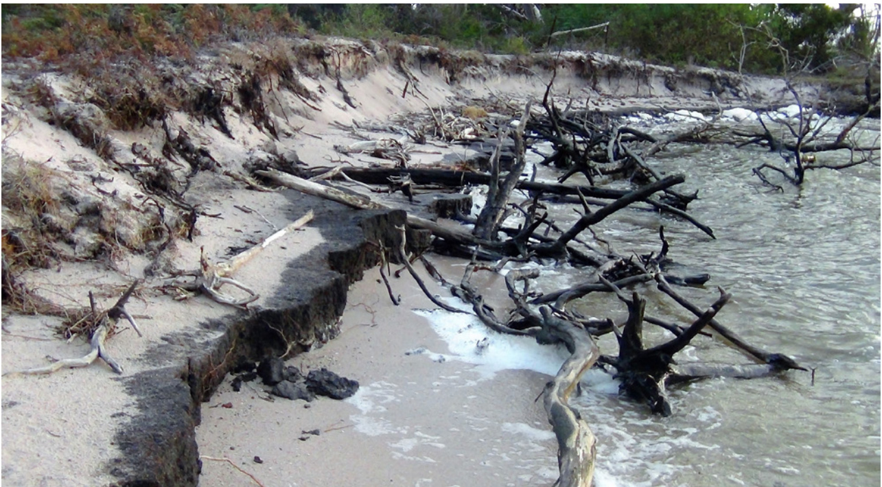
Figure 9 – Erosion of foreshore at eastern end of Wellington Park
