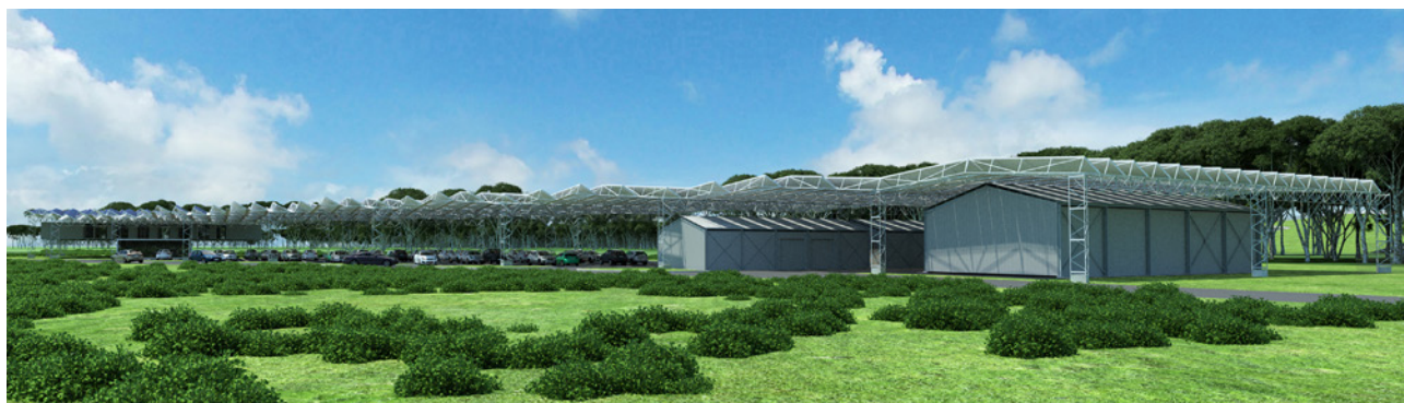
Figure 37 – Indicative image of the infrastructure area looking north-west
