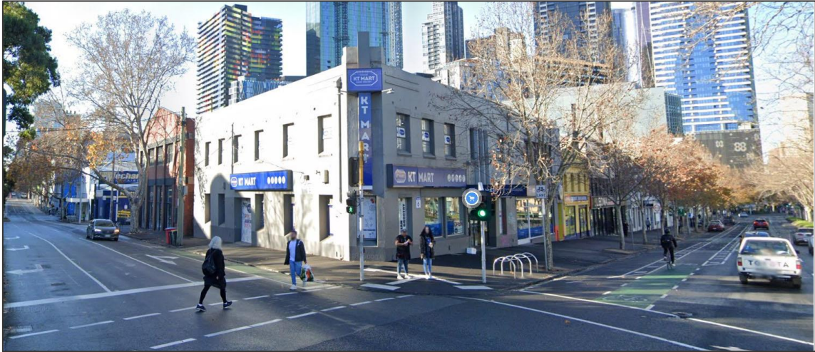
Figure 4: Subject site from corner of Elizabeth and Queensberry Street (Source: Google Maps)
