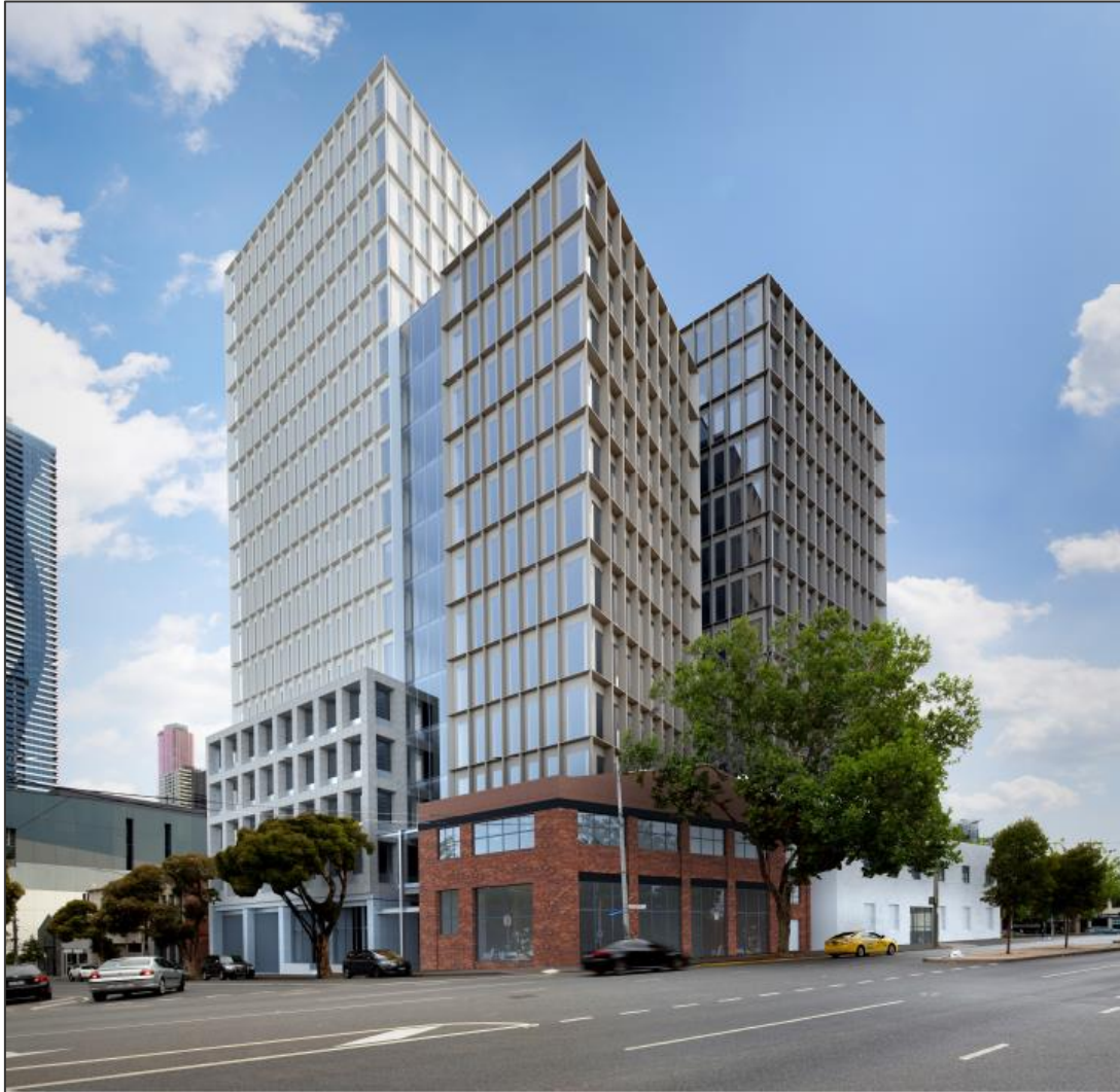
Figure 10: Concept image of proposal from the north east corner of Queensberry and Berkeley Streets (Source: Application)
