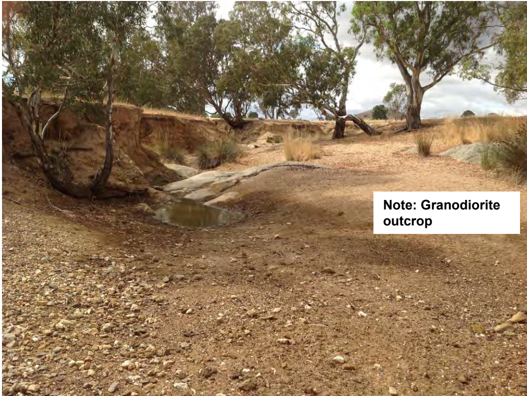
PHOTOGRAPH 5 – Erosion Washout in Granitic soils
