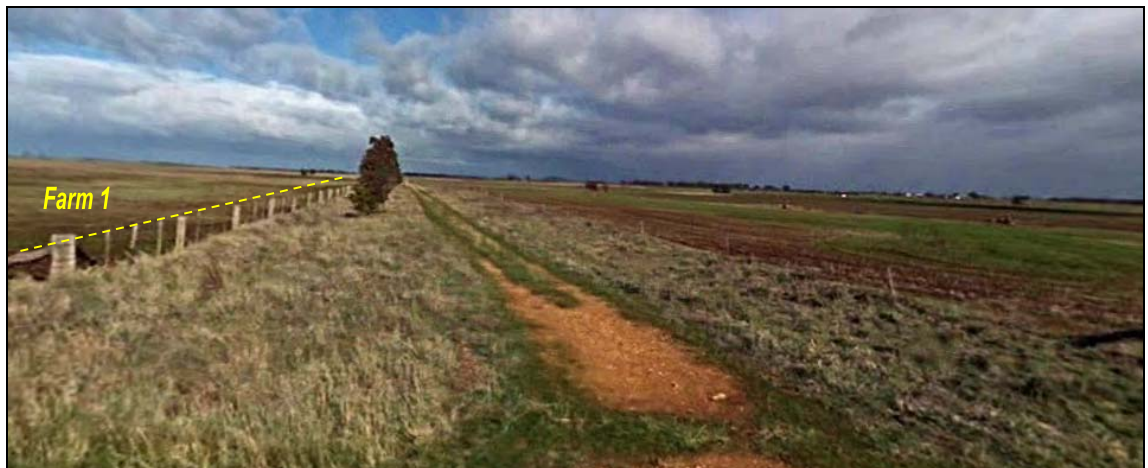
Figure 5: O'Keefes Road Reservation Looking South from Baringhup West Road
