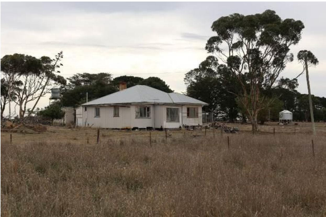
FIGURE 52 – RESIDENCE 89 ON VEALS LANE (DERELICT HOUSE IN FRONT OF MAIN RESIDENCE) – CHARACTER OF SETTING
