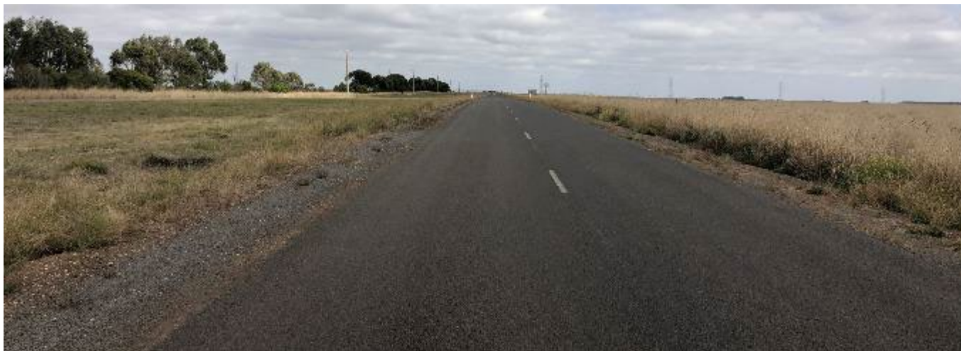
Figure 8 Darlington-Terang Road looking south, approximately 140 metres south of Hamilton Highway
