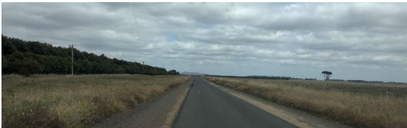
Figure 9 Darlington-Terang Road looking south, approximately 6.9 km south of Hamilton Highway
