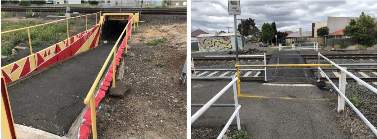
Figure 6-5: Barwon Avenue underpass and Drake Street level crossing
