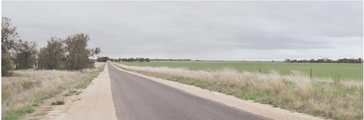
Figure 51 VP21 looking north east along the Borung Highway
