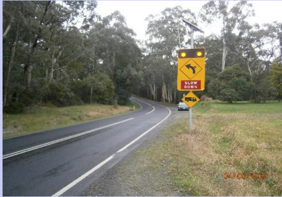
Dalry Road Warning Sign with One Light Displaying Continuously
