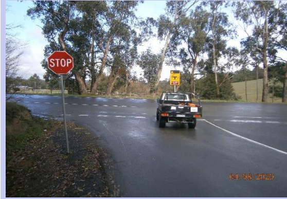
Incorrect 'Give Way Hold Line' Marking at Intersection
