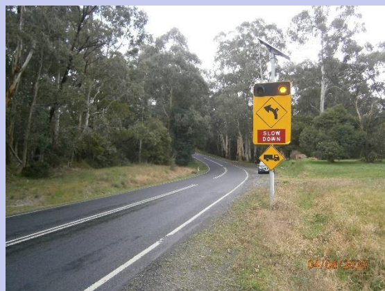
Advance Warning Sign on Dalry Rd East Approach
