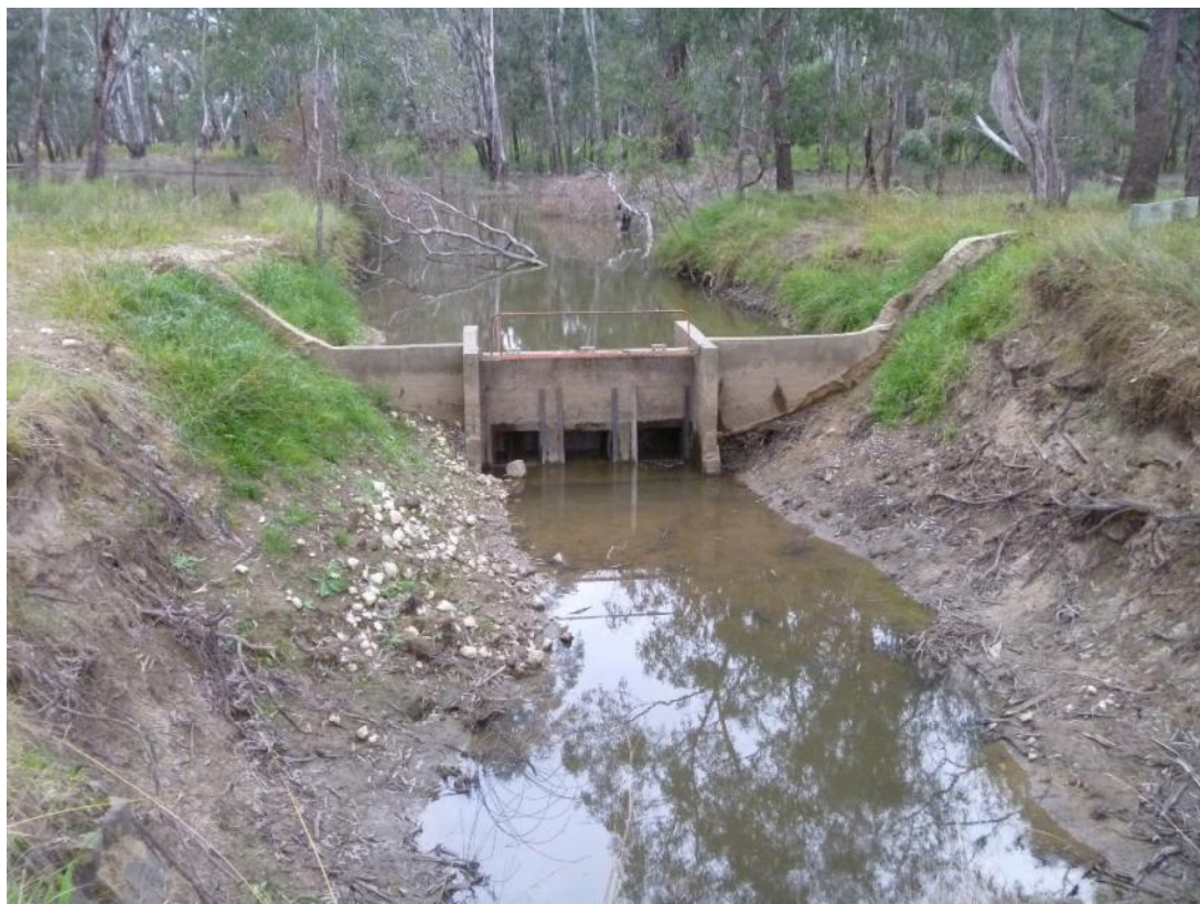
Figure 3-8 Water level downstream of the Lake Moodemere regulator on 8 July 2011 with Murray River flow of 12,200 ML/D at Corowa or 11,400 ML/D at Doctors Point
