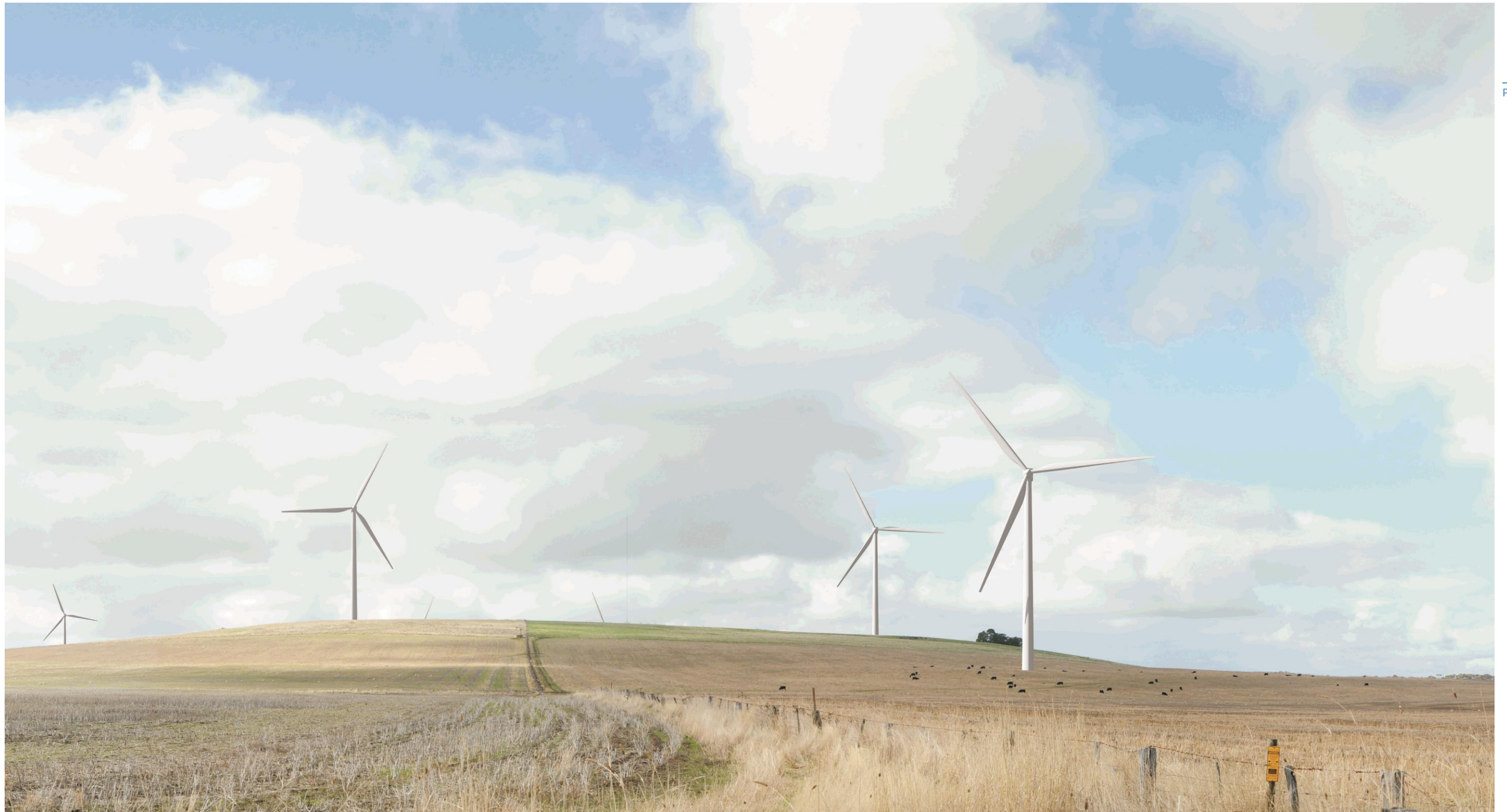
Figure 7-7 Viewpoint N03 – 60 degree views of the Permitted WEF (above) and the Amended WEF (overleaf) looking east
