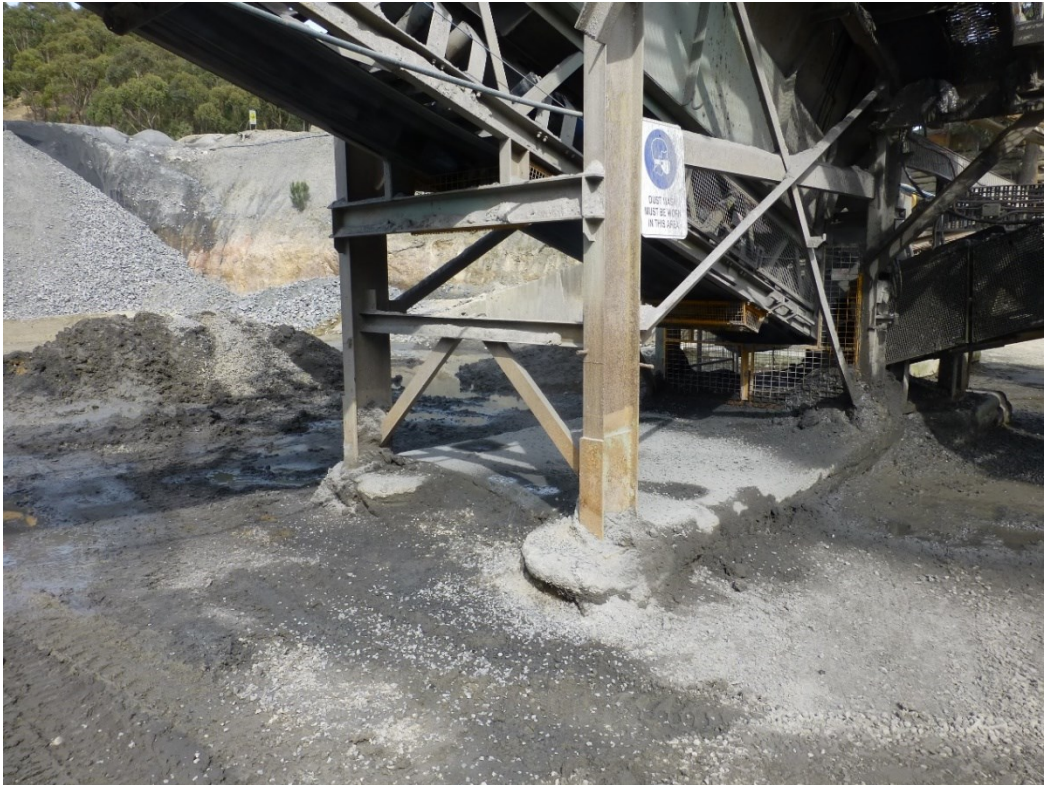
Figure 5. The dust sample was collected from the lower, horizontal beam on the 18 mm screen's support structure
