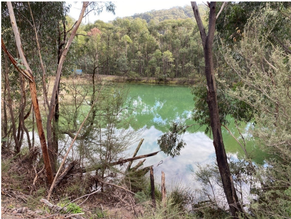
Figure 4. Photograph of Main Dam
