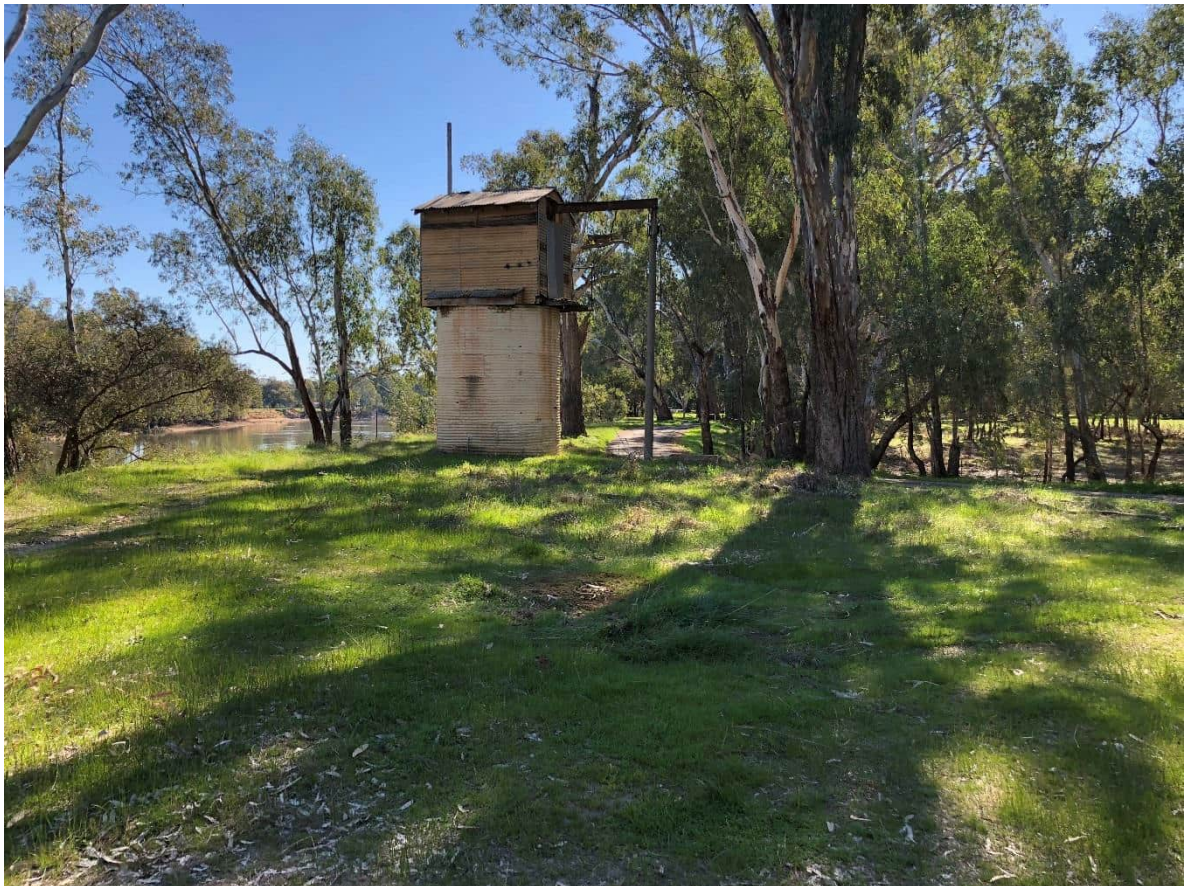
Photo 2: Existing site conditions – Site 2, Pump Station.
