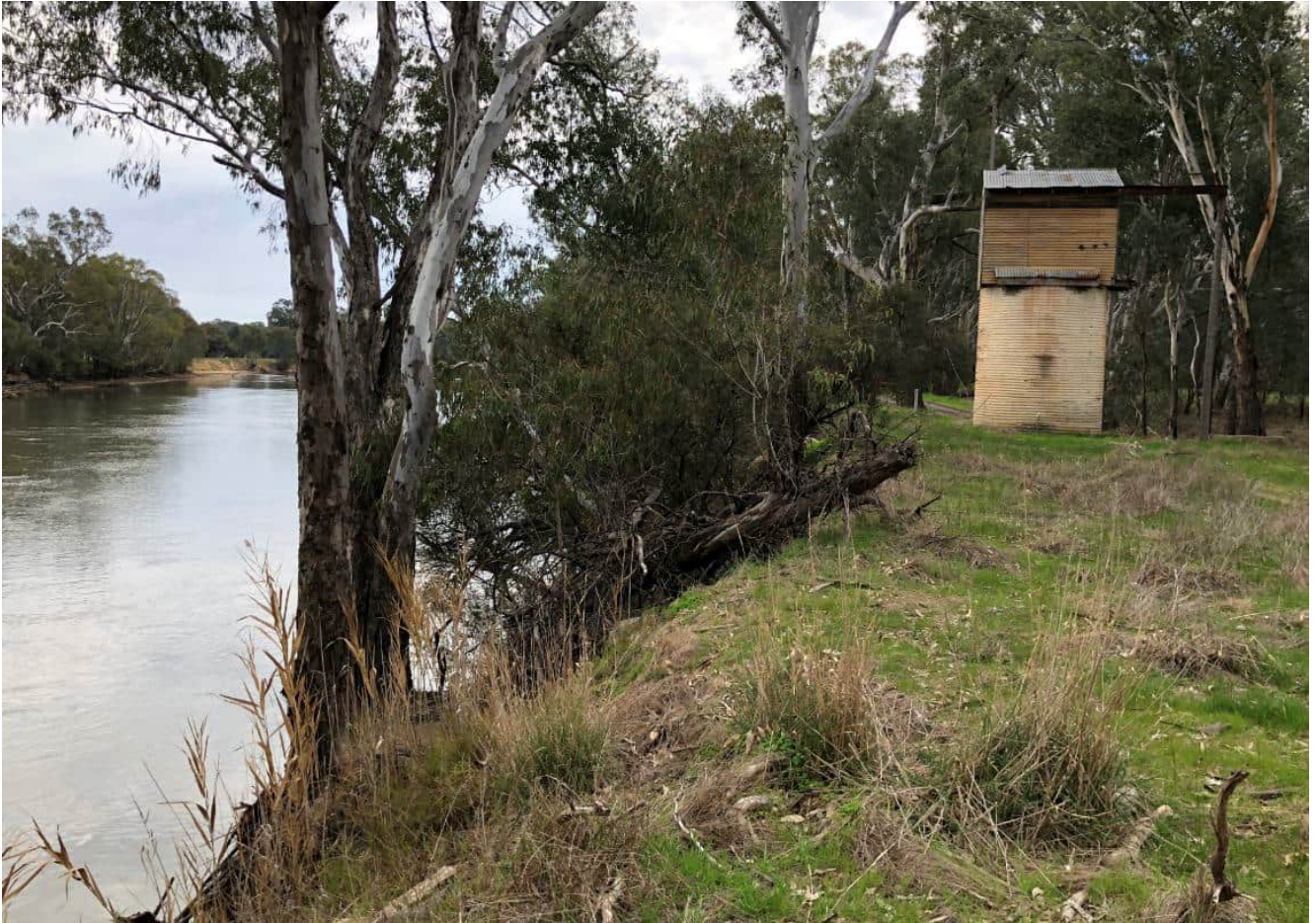
Figure 4-2: Sunday Creek River Pump Station Location
