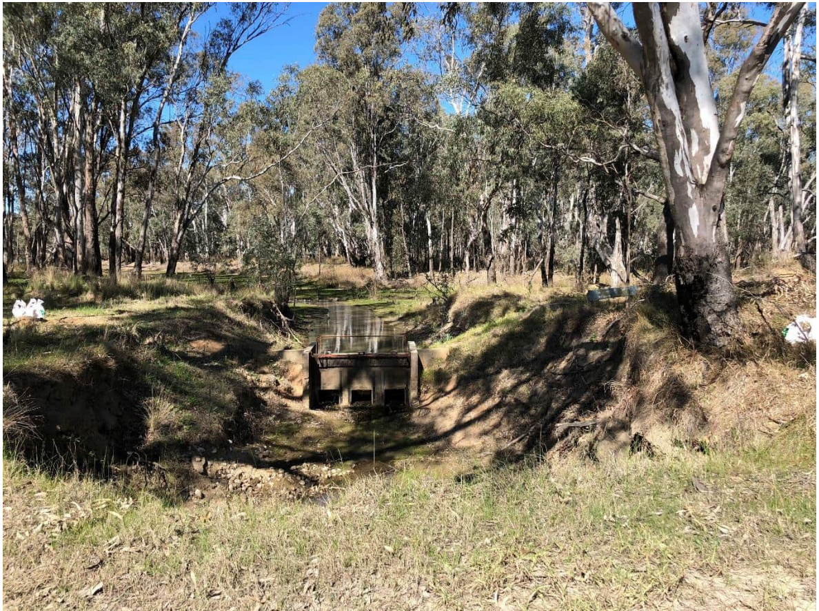
Photo 1: Existing site conditions – Site 1, Regulator.
