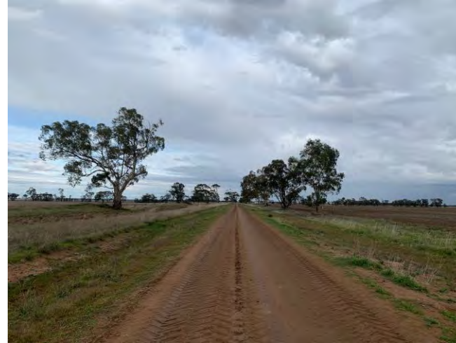
Photograph 10: Dogwood Road View South
