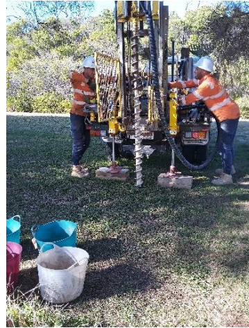
Photo 2: Set-up over Borehole 7.
