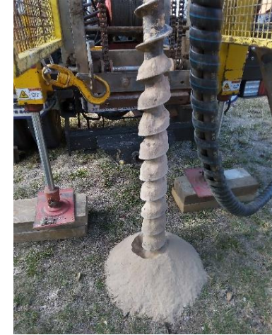
Photo 3: Auger spoil material from Borehole 7.
