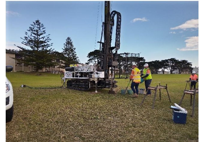
Photo 3: Location of borehole 1
