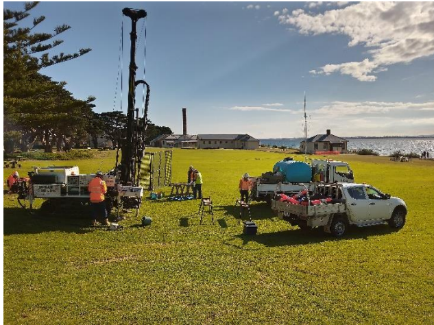
Photo 8: Location of borehole 2.
