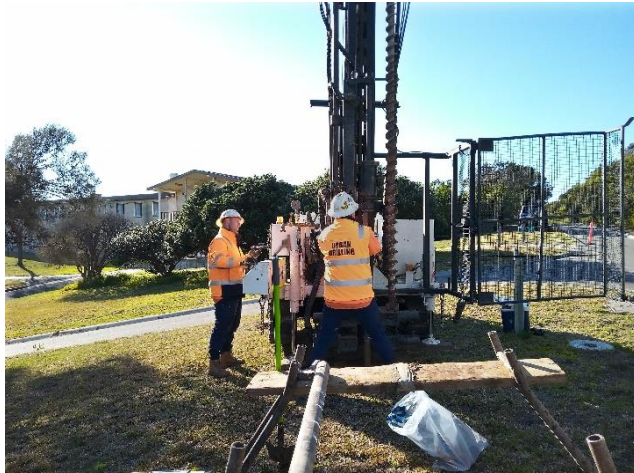
Photo 17: Location of borehole 4.
