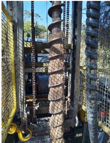
Photo 11: Excavated soil material from Borehole 8.
