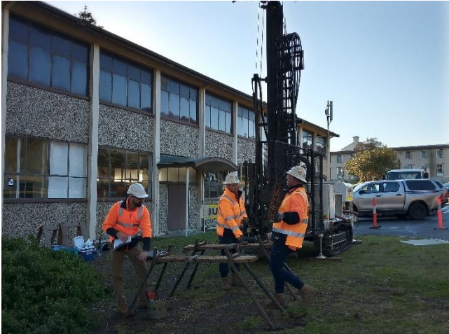
Photo 13: Location of Borehole 3.
