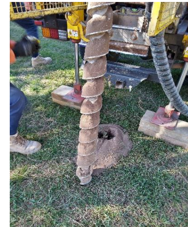
Photo 6: Excavated soil material form Borehole 7.
